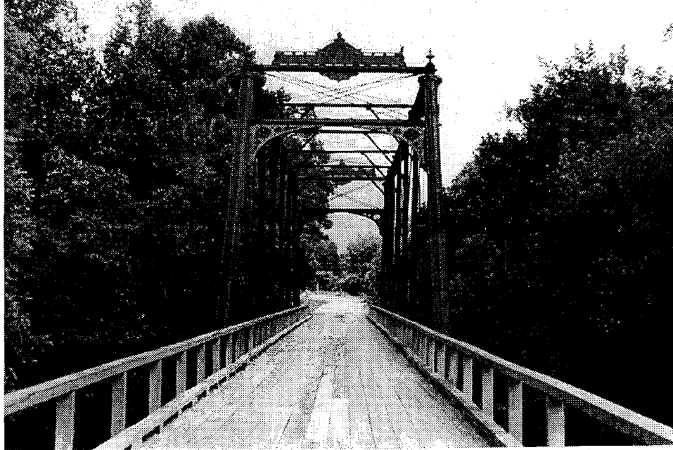
Figure 10. Highly Ornamental Pratt Through Truss with Phoenix Columns Built in 1887 (Botetourt County Structure No. 6386)
