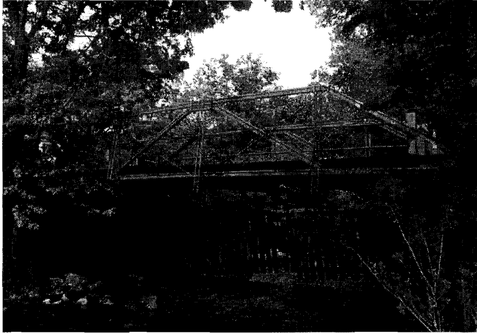
Figure 6. Lane Patent Pony Truss, Built in 1896 (Highland County Structure No. 6034)
