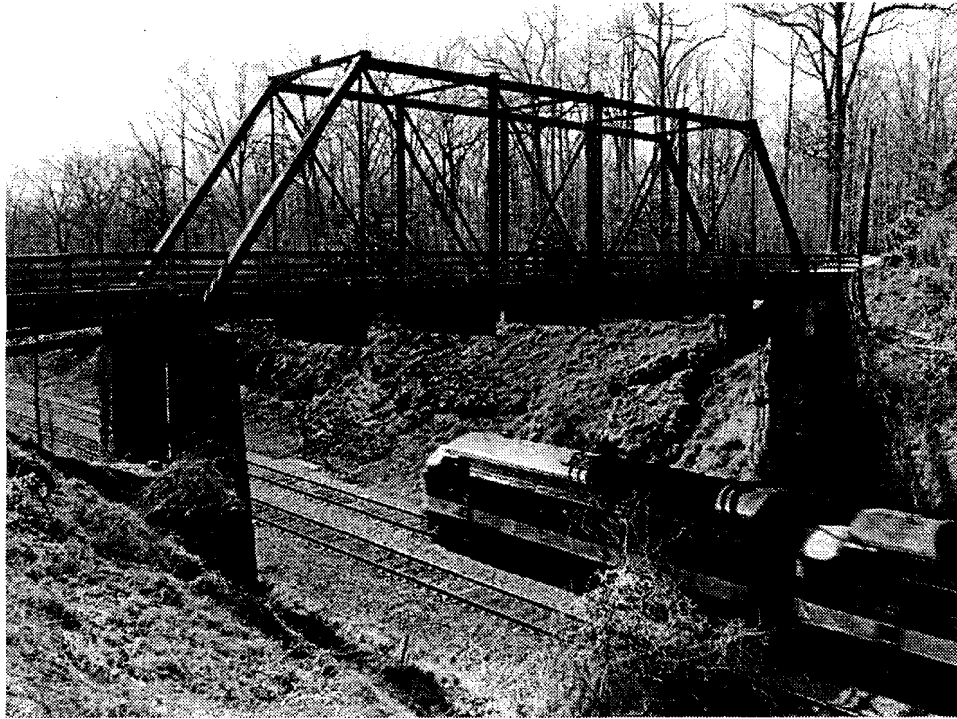
Figure 12. Pratt Through Truss Built in 1882 (Nelson County Structure No. 6052)
