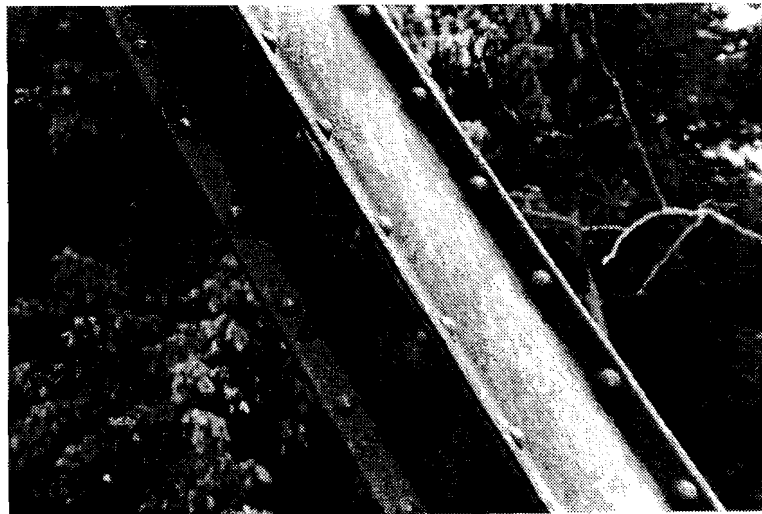
Figure 4. Detail of Patented Phoenix Column (Botetourt County Structure No. 6386)
