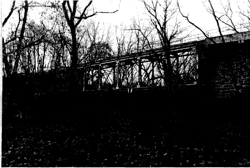
Figure 9. Pratt Deck Truss. Truss built in 1915 on Virginia & Tennessee Railroad stone abutments built around 1850 (Bedford County Structure No. 6087)
