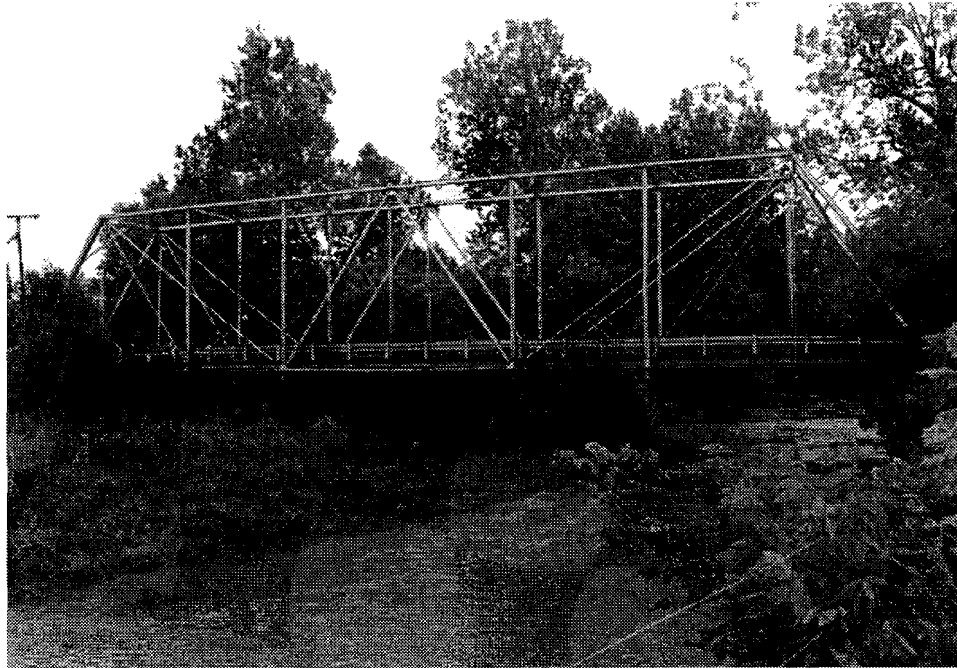
Figure 7. Thatcher Truss Built in 1898 (Rockingham County Structure No. 6154)
