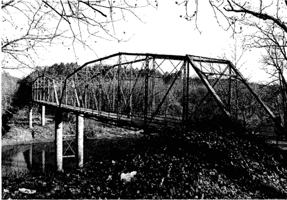
Figure 11. Camelback Through Truss Built Around 1900 (Charlotte County Structure No. 6902)
