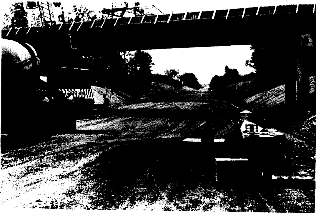
Figure 2. View of concrete discharge, sampling and testing area on B 648. One 3/4 yd 3 bucket is filled and waiting for the return of crane, which has just completed discharge on the deck.
