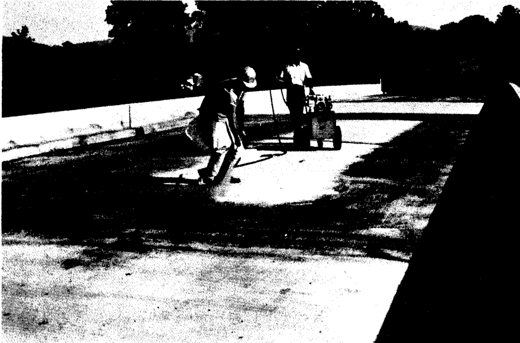
Figure 9. LOT treatment on Span 3 of B 648. In the foreground is CRS panel. The LOT is being applied to Panel 1, cured with LMS, with no additional treatment to remove the LMS.
