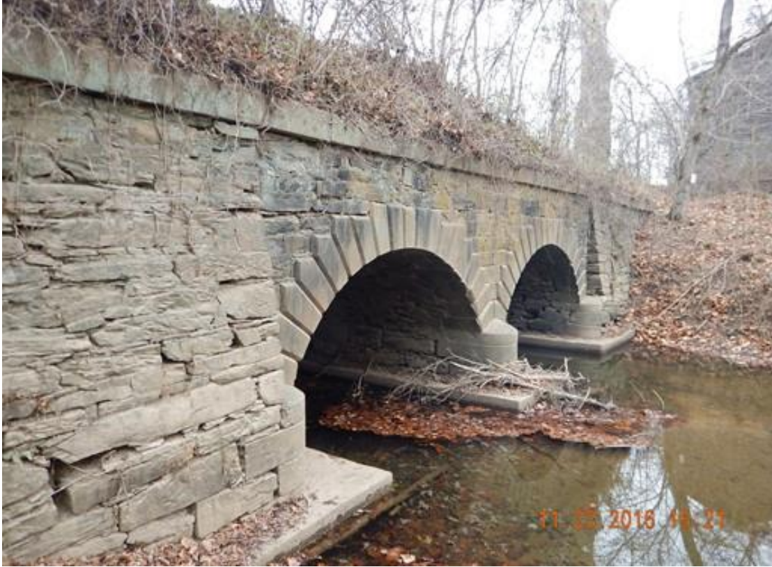
Figure 4. Stone Masonry Arch, Originally Built as a Canal Viaduct, 1835 (Nelson County Structure No. 6070). Note the particularly fine finishing of the voussoirs.
