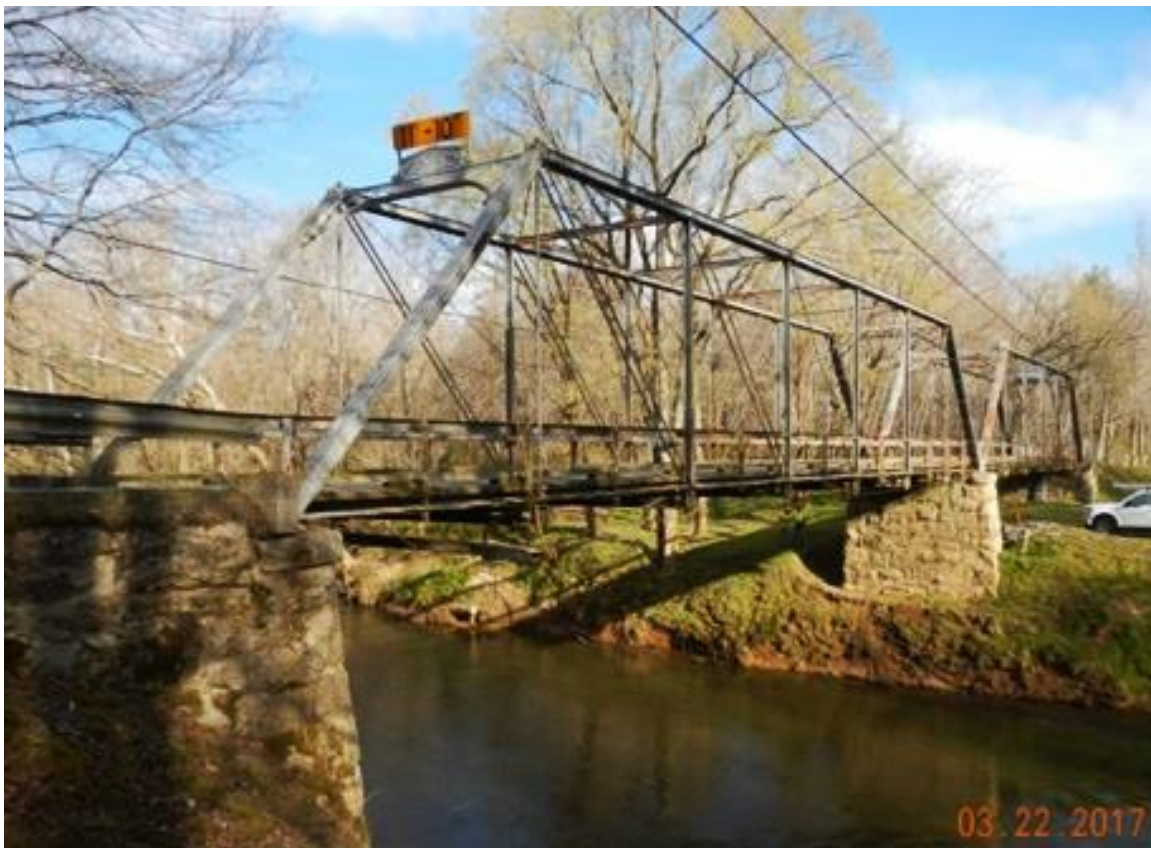
Figure 1. Stone Masonry Piers and Abutments Supporting an 1884 Truss Bridge (Brunswick County Structure No. 6104)
