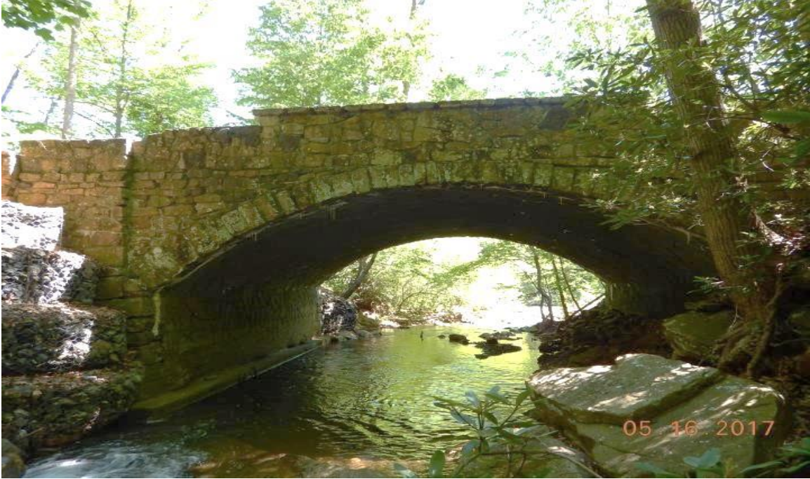
Figure 6. Stone Masonry Veneer on a Concrete Bridge in a Rustic Setting, 1940 (Rockbridge County Structure No. 1012)
