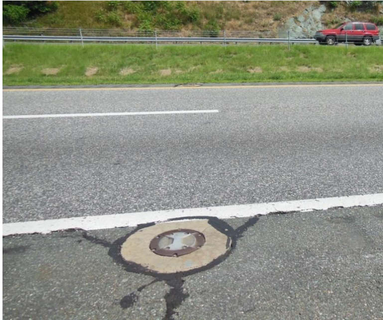
Figure 7. Fog Lights on I-64 Over Afton Mountain
