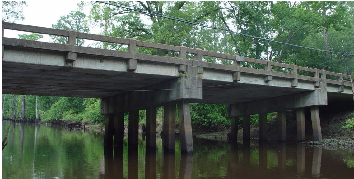
Figure 23. Side View of Adkins Road Bridge
