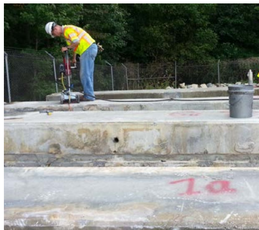
Figure 6. Beams of Qualla Road Bridge Placed Upside Down in VDOT Yard
