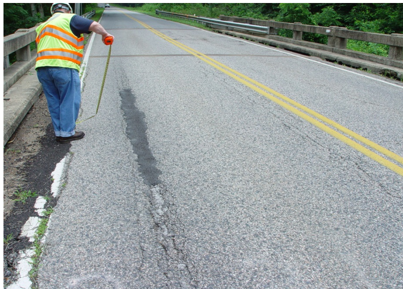
Figure 13. View of Deck of Qualla Road Bridge Over Swift Creek
