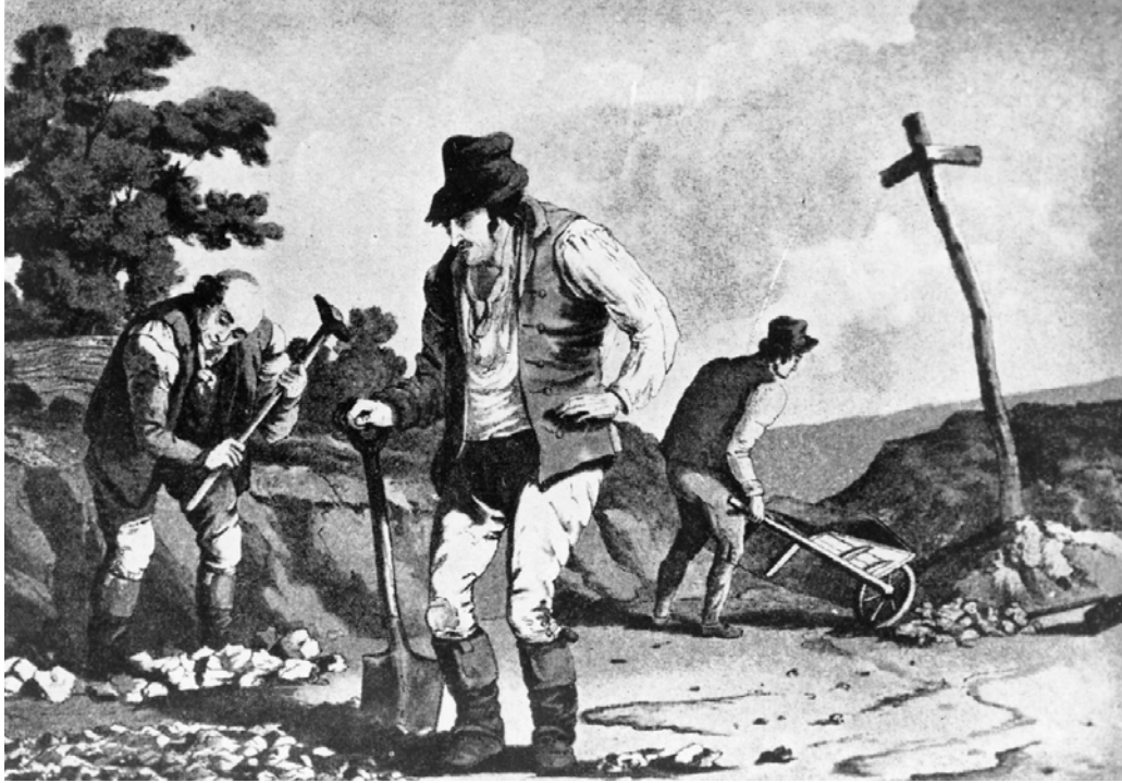
Early Virginians were required to help with the construction and maintenance of the roads. [NOTE: This early 19 th century engraving shows road workers in Yorkshire, England, but similar scenes would have occurred elsewhere in Great Britain, in Europe, and in the United States; from George Walker, “Stone-Breakers on the Road,” from his series Costume of Yorkshire , 1814.]
