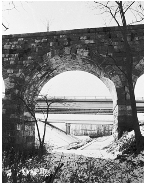
Railroad bridge on Interstate 81 four miles south of Staunton.
