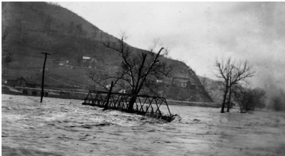
A metal truss bridge over the James River in Alleghany County is overcome by the rising waters during a 1936 flood.
