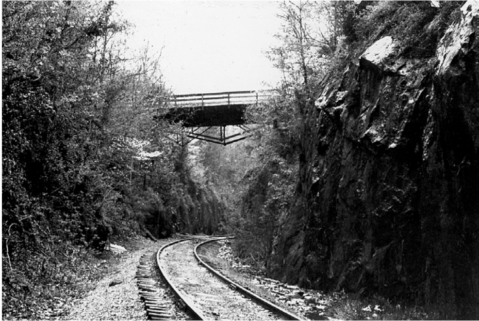
The Fink Truss [NOTE: in its 1890s location on Route 291 (Old Forest Road)].
