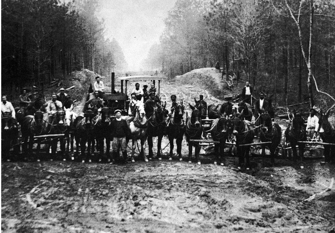
Men and mules supplied labor for building state roads in the early 1900s.
