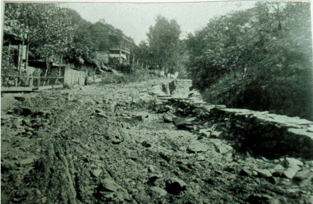
“Section of road in Amherst County before improvement.”
