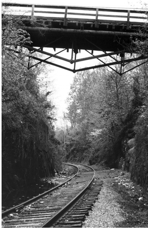
The Research Council is now making an inventory of the state's metal truss bridges. [NOTE: This is the Virginia Fink truss described in the article.]
