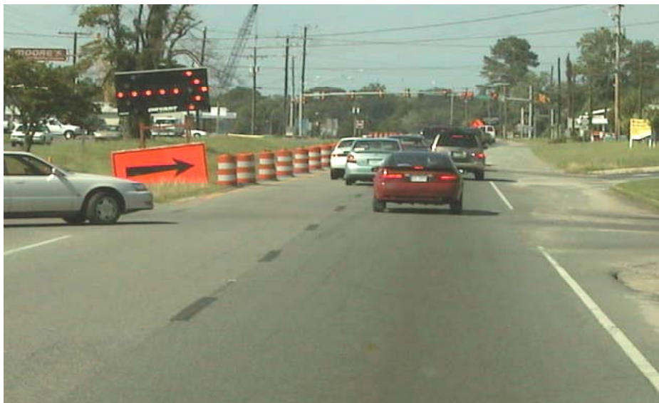
Figure 19. Tappahannock Lane Closure
