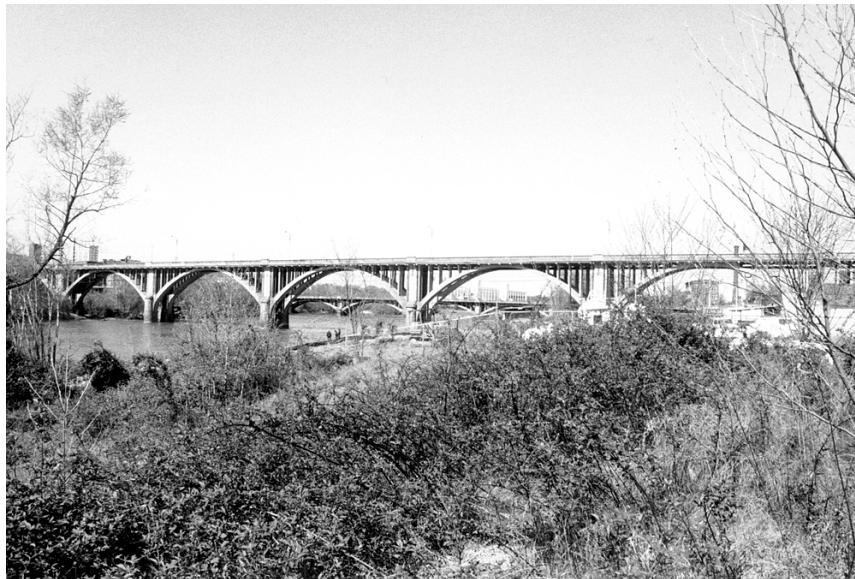
Figure 15. Open Spandrel Concrete Arch, a Luten Bridge Company Design Built in 1928 (City of Danville Structure No. 8006)
