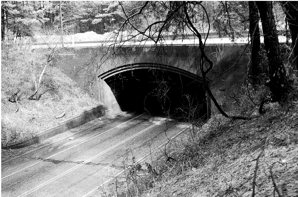
Figure 19. Concrete Rigid Frame with Brick Veneer, a U.S. Department of Public Roads Design, Built in 1936 at the Petersburg National Military Park (City of Petersburg Structure No. 8018)
