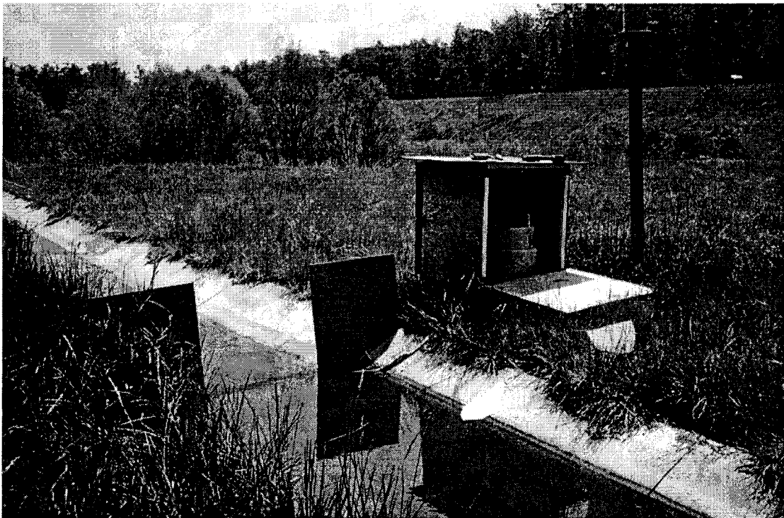
Figure 2. Typical monitoring station (Rt. 288 infow)
