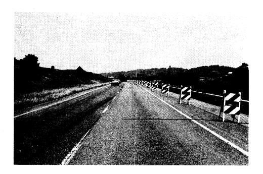
Figure A-2. Type II barricade with 6-in. (15.2-cm) stripes.
