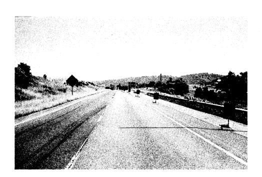
Figure A-6. Chevron with a black arrow - 80-ft. (24.4-m) taper spacing.
