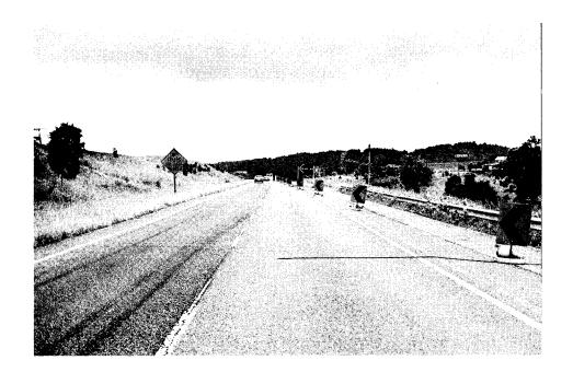
Figure A-8. Large chevron with black arrow — standard mount with 80-ft. (24.4-m) taper spacing.
