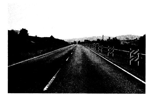
Figure A-1. Type II barricade with 4-in. (10.2-cm) stripes.
