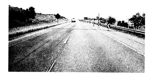
Figure A-4. Chevron with a white arrow - 40-ft. (12.2-m) taper spacing.
