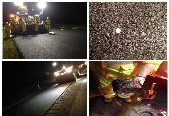
Figure 8. Placement of AR-GGM Mixture
