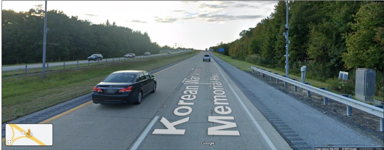
Figure 18. Google Street View Image of APRS on State Route 1 in Delaware
