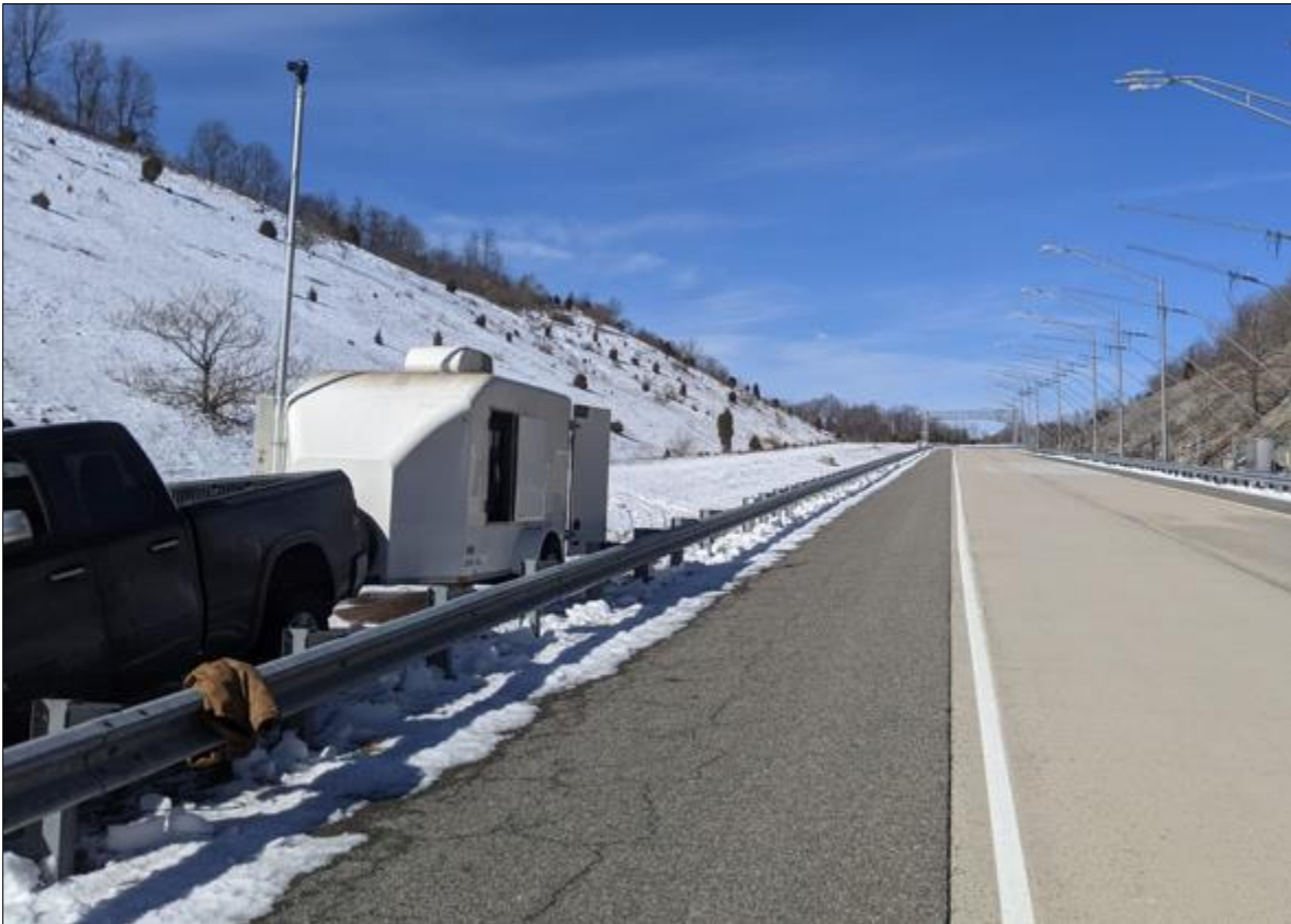
Figure 9. View of the APRS Trailer Configuration Used for Virginia Smart Roads Testing
