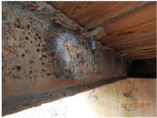
Figure 15. Example of Steel Beam Timber Deck Web Corrosion
