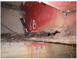
Figure 1. Example of Extensive Beam End Corrosion Damage
