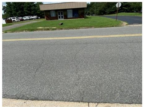
Figure 15. FDR + 2.5-in AC Surface on Lee Park Road, 8 Years After Construction. FDR = full depth reclamation; AC = asphalt concrete.
