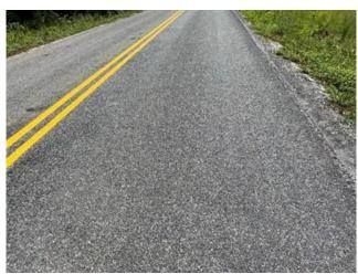
Figure 10. FDR + Blotted Seal Coat, 1.5 Years After Construction. FDR = full depth reclamation.
