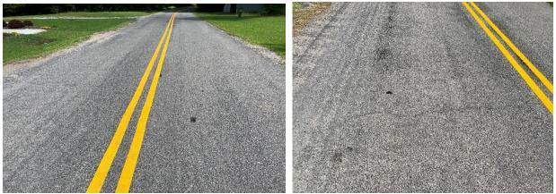
Figure 9. FDR + Modified Double Seal Layer, 1.5 Years After Construction. FDR = full depth reclamation.
