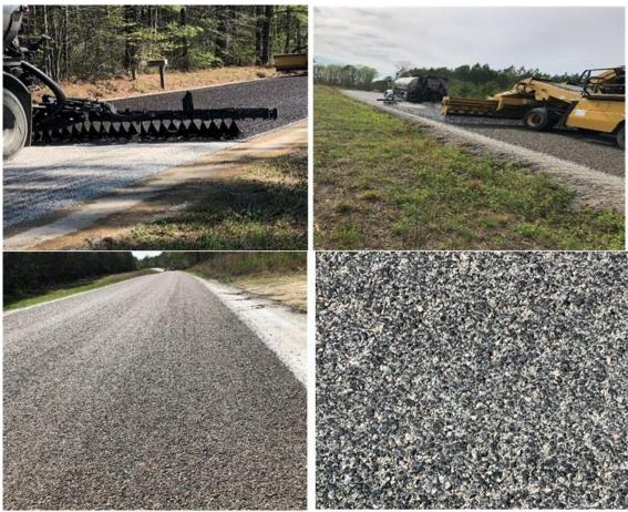
Figure 7. Blotted Seal Placement on Rte. 602 FDR. FDR = full depth reclamation.
