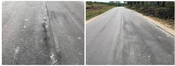
Figure 4. Segregation and Raveling on SM-9.0 Mix Placed Over Second FDR Trial. FDR = full depth reclamation.
