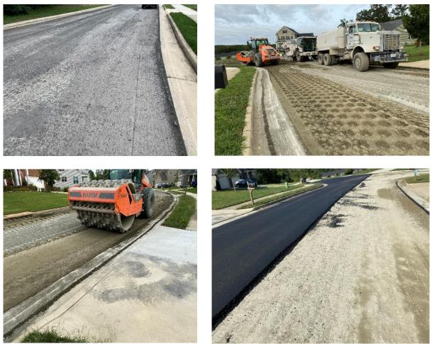
Figure 8. FDR and Asphalt Paving at Estates at Leeland. FDR = full depth reclamation.
