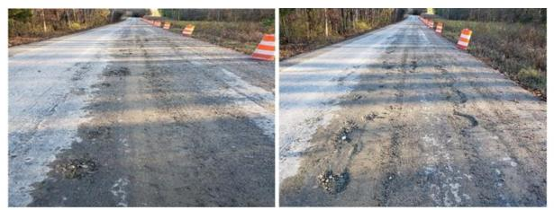
Figure 3. First FDR Trial Section on Rte. 602. FDR = full depth reclamation.
