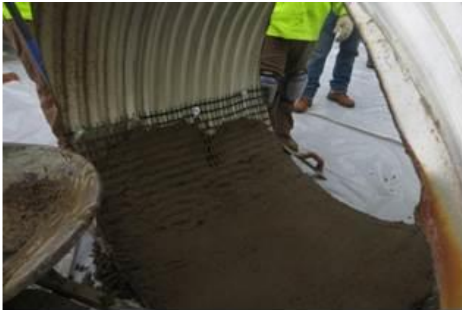
Figure 10. ECC From Trial Batch Flowing Down Sides in Ripples. ECC = engineered cementitious composite.
