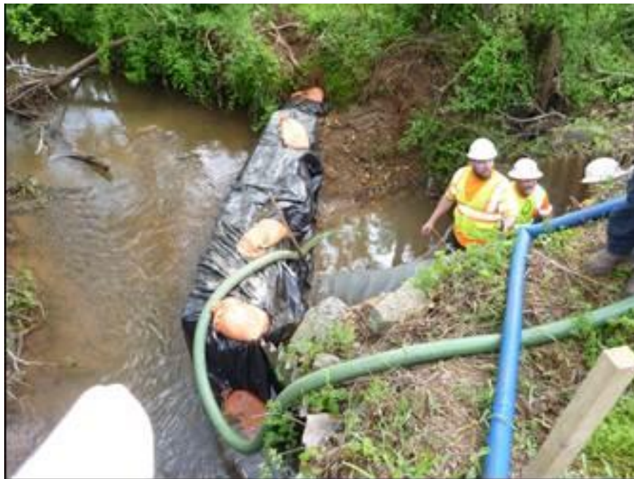
Figure 2. Dewatering
