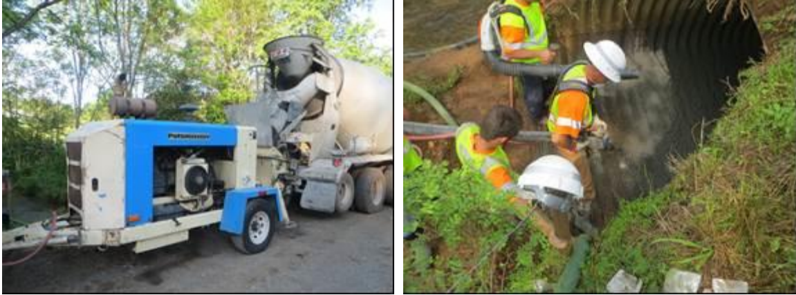
Figure 4. Trailer Pump (Left), Spraying Engineered Cementitious Composite (Right)
