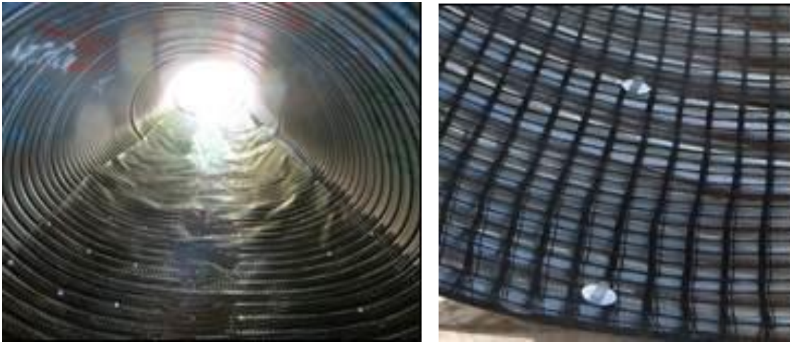
Figure 3. Geogrid Attached (Left), Screw With Spacer (Right)
