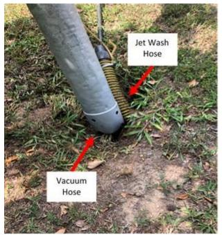
Figure 4. Clean-out of the Driveway Pipe Shown in Figure 3. Here the jet wash hose is used to loosen and flush out material although the vacuum hose collects it.
