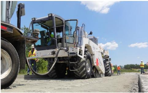
Figure 1. Reclaimer Used for Full Depth Reclamation
