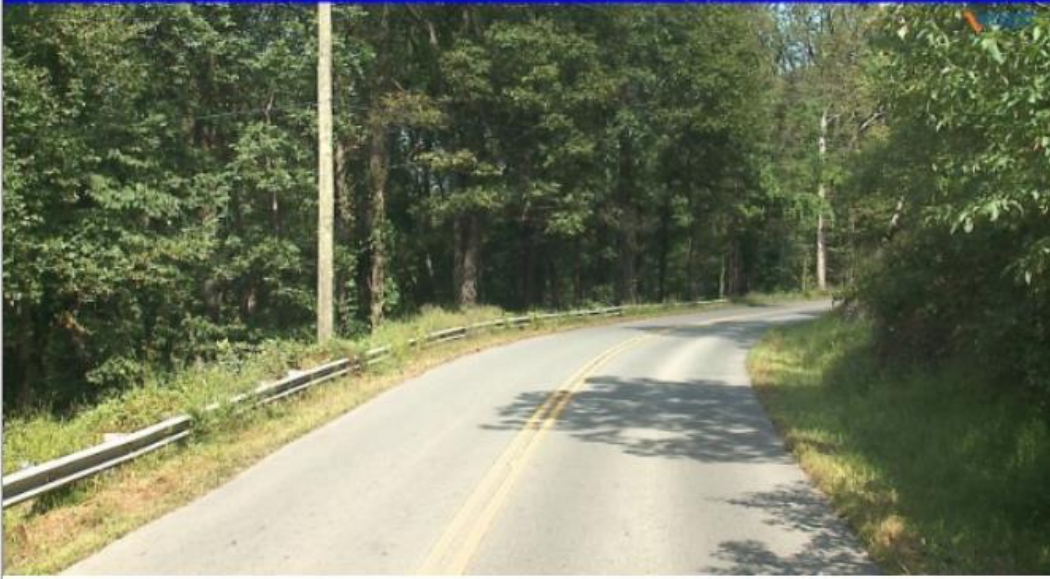
Figure 13. Segment Near MP 6.52
