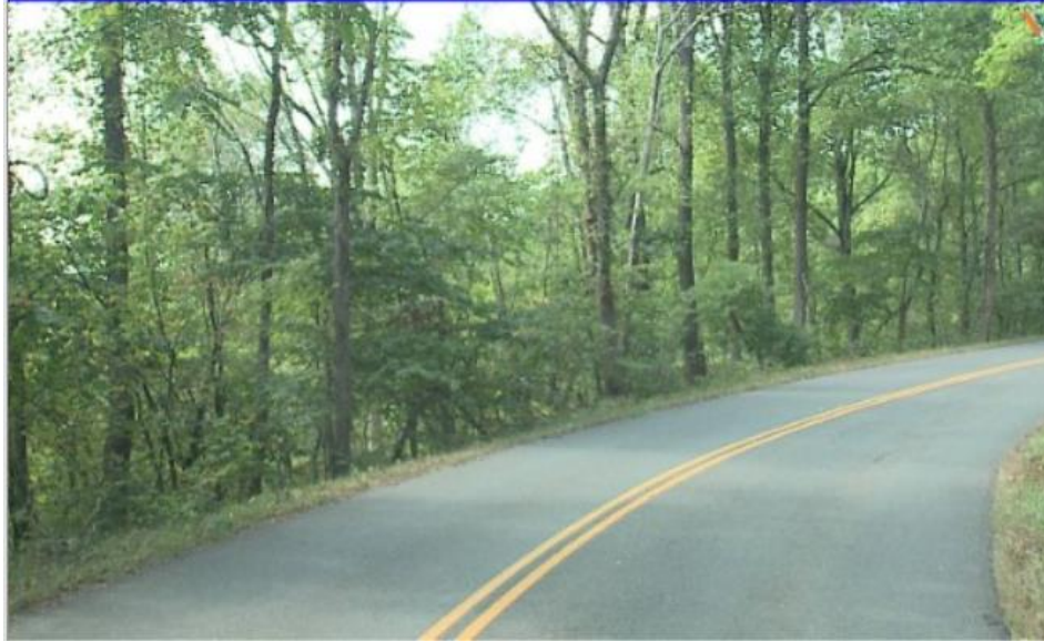
Figure 15. Segment Near MP 2.57
