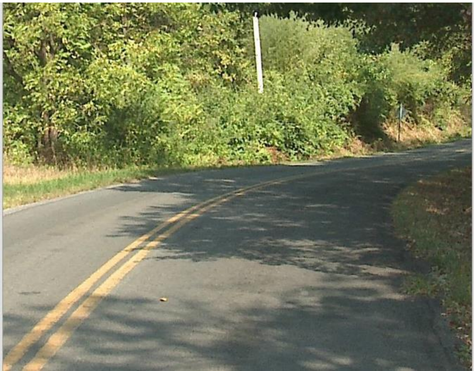
Figure 14. Segment Near MP 12.71
