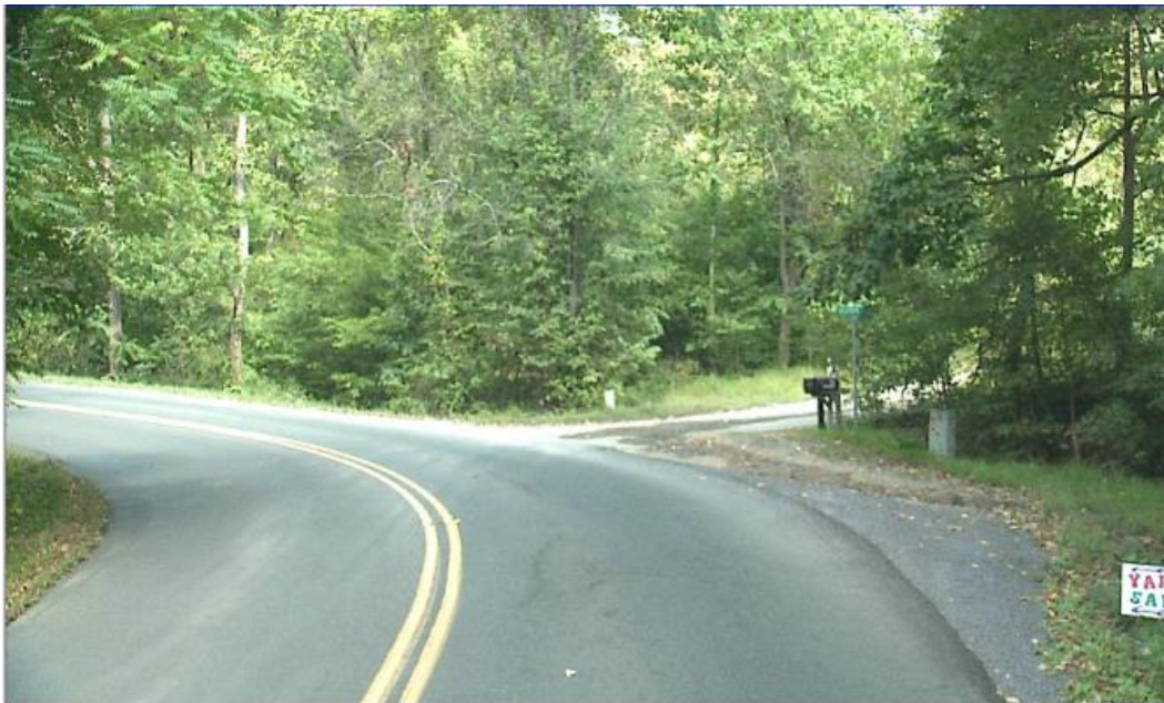
Figure 12. Segment Near MP 2.45
