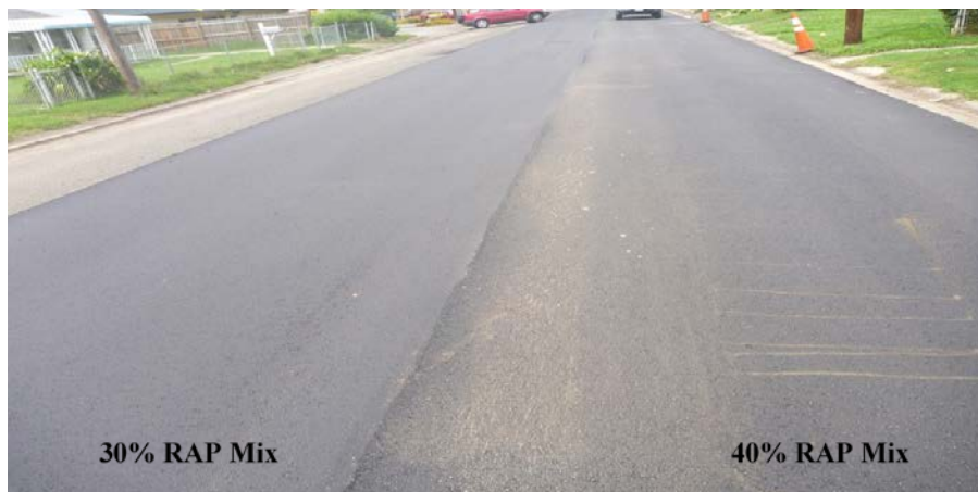
Figure 2. Final Pavement Surface at Sherdon Street. RAP = reclaimed asphalt pavement.
