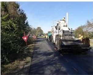
Figure 11. Interlayer and Overlay Placement on SR 30
