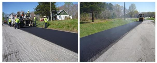
Figure 4. Asphalt Overlay Placement
