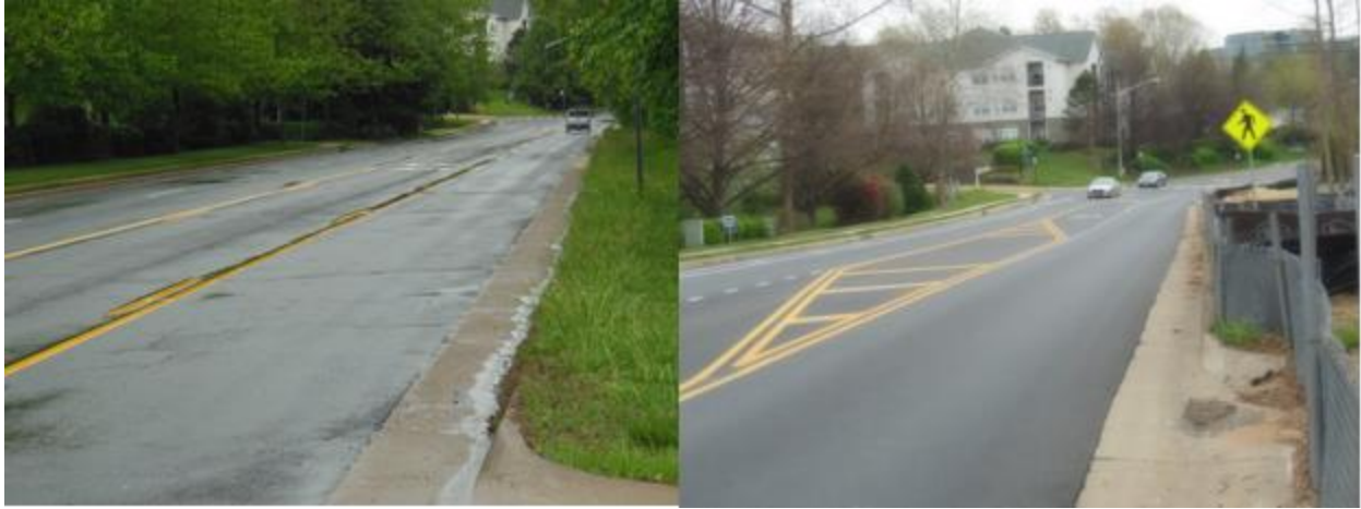
Figure 8. Before (Left) and After (Right) Photographs of Road Diet on Post Forest Drive
