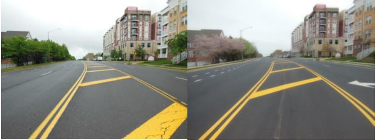
Figure 10. Before (Left) and After (Right) Photographs of Road Diet on Ridge Top Road Between Government Center Parkway and Lee Highway
