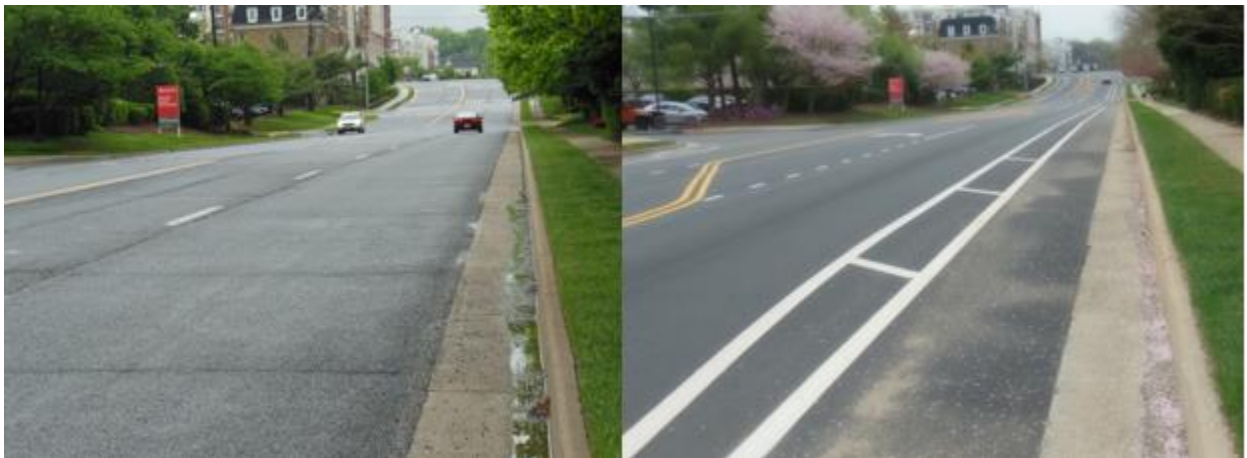
Figure 9. Before (Left) and After (Right) Photographs of Road Diet on Ridge Top Road Between Random Hills Road and Government Center Parkway
