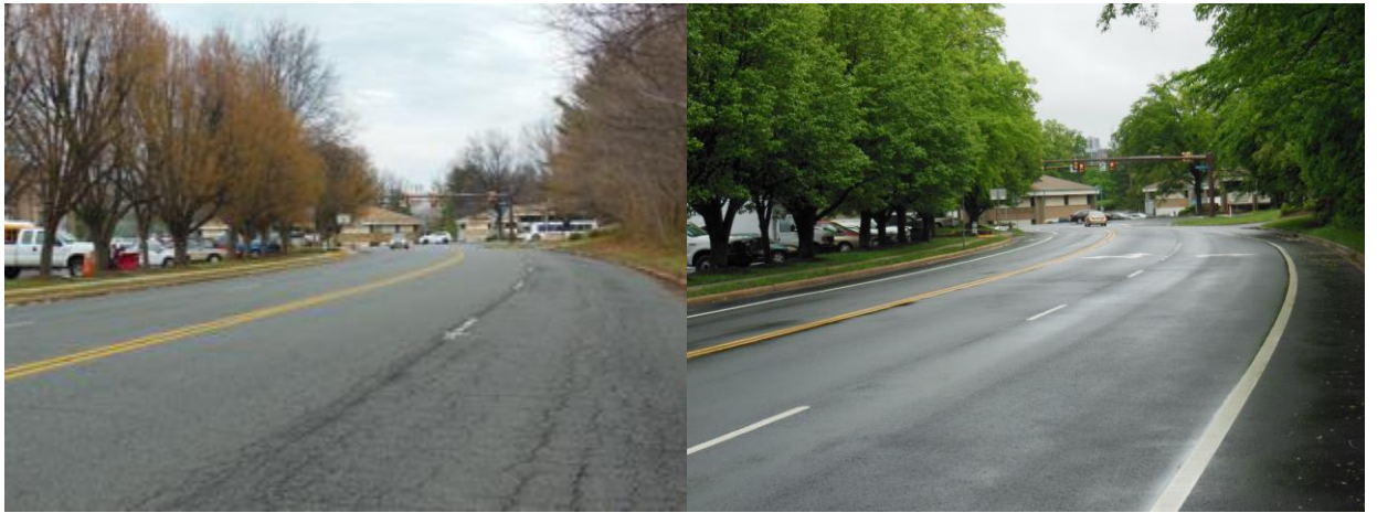
Figure 7. Before (Left) and After (Right) Photographs of Road Diet on Colts Neck Road, Northern Segment
