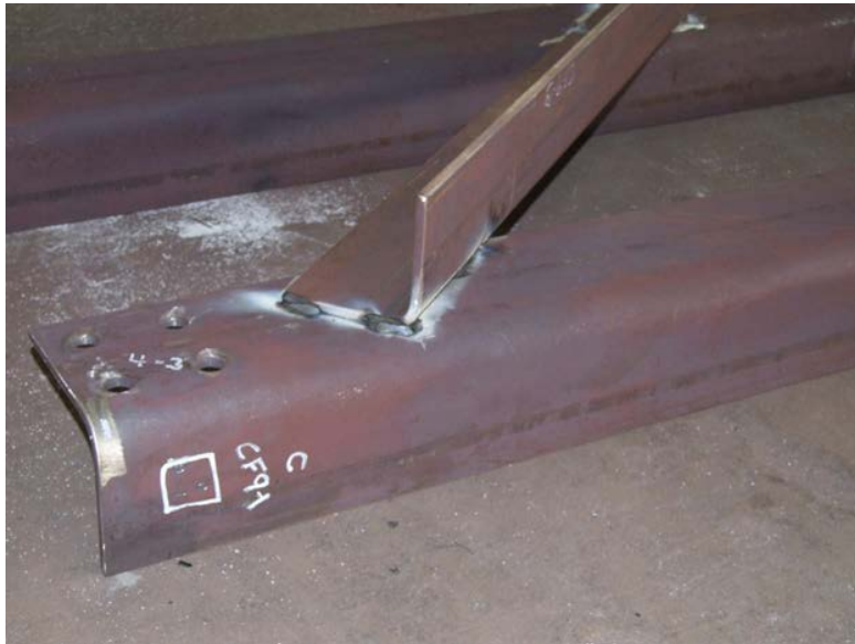
Figure 14. Close-up of A1010 Steel Bent Plate Cross Frame With Welded Connection
