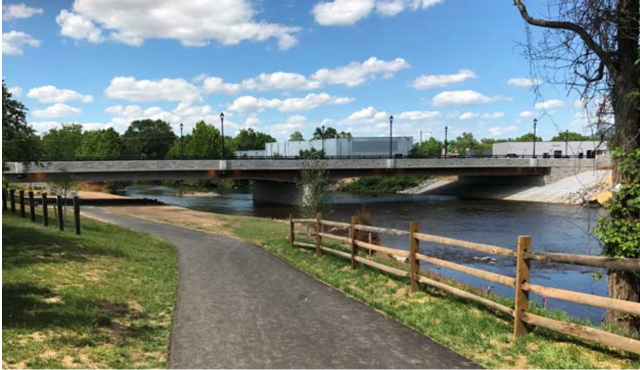
Figure 27. Award-Winning Route 340 Bridge in Waynesboro, Virginia
