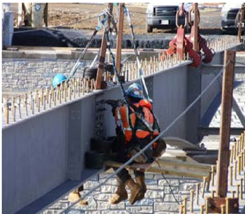
Figure 25. Installation of Stainless Steel Fasteners on Bolted Splice
