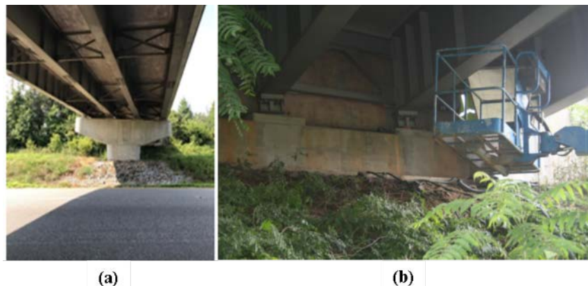
Figure 5. On-site Demonstration of LACR: (a) underside of Route 695 Bridge in Farmville, Virginia, where the on-site LACR testing took place; (b) boom lift used to elevate the operator to the cleaning area. LACR = laser ablation coating removal.
