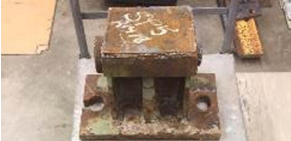
Figure 6. Bridge Bearing Component Used in Phase 3
