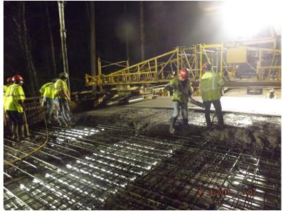
Figure 5. Bridge Construction Showing Nighttime Deck Concrete Placement
