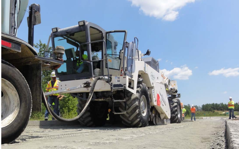
Figure 1. Reclaimer Used for Full Depth Reclamation
