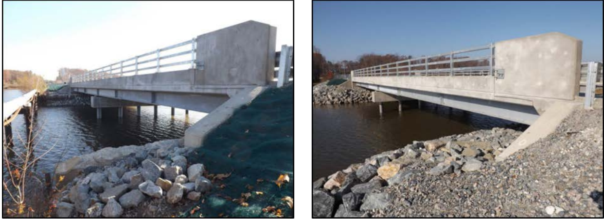
Figure 9. Images of the Genito Road Bridge From the Initial VDOT Inspection Report in 2012: left, upstream (north) elevation; right, downstream (south) elevation
