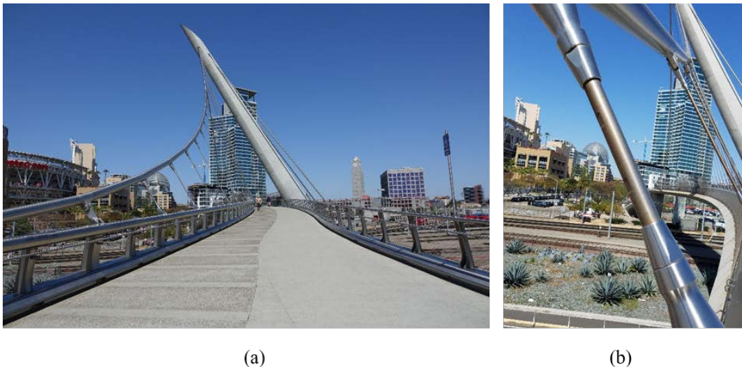
Figure 27. Harbor Drive Pedestrian Bridge: (a) overall view; (b) close-up of Grade 2205 duplex stainless steel suspender. Photograph courtesy of Catherine Houska.
