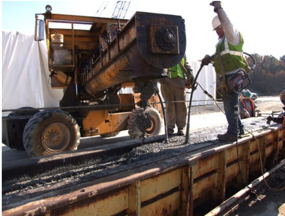
Figure 7. Concrete Consolidation Using Rubber Tipped Vibrators
