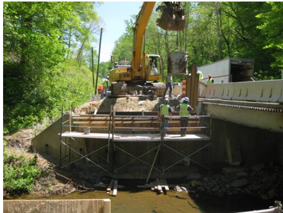
Figure 1. Bucket Being Used to Place Concrete Into Backwall for Route 699 Bridge
