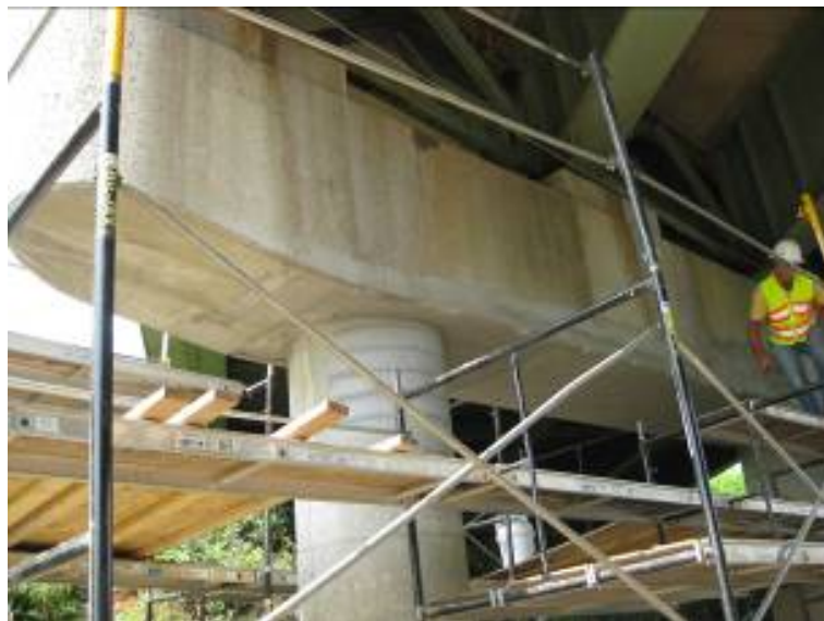
Figure 12. Repaired Cap and Column of Route 712 Bridge
