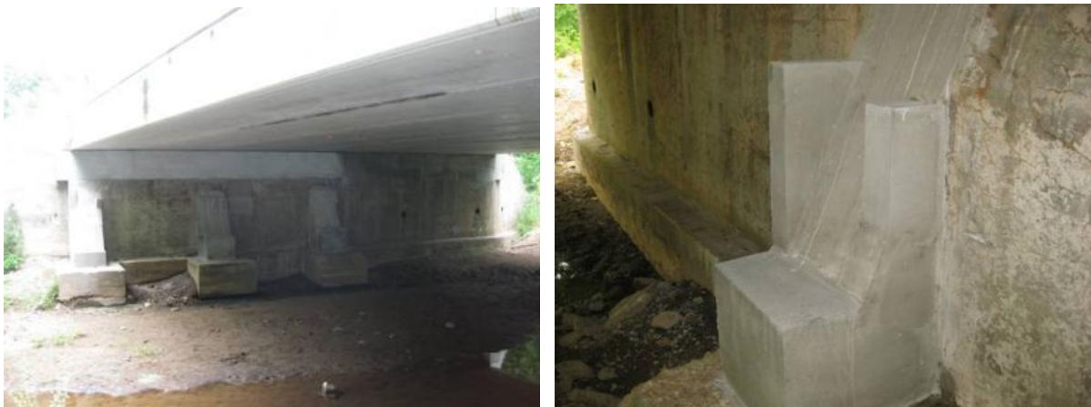
Figure 9. SCC Repaired Backwall ( left ) and Buttress ( right ) for Route 699 Bridge
