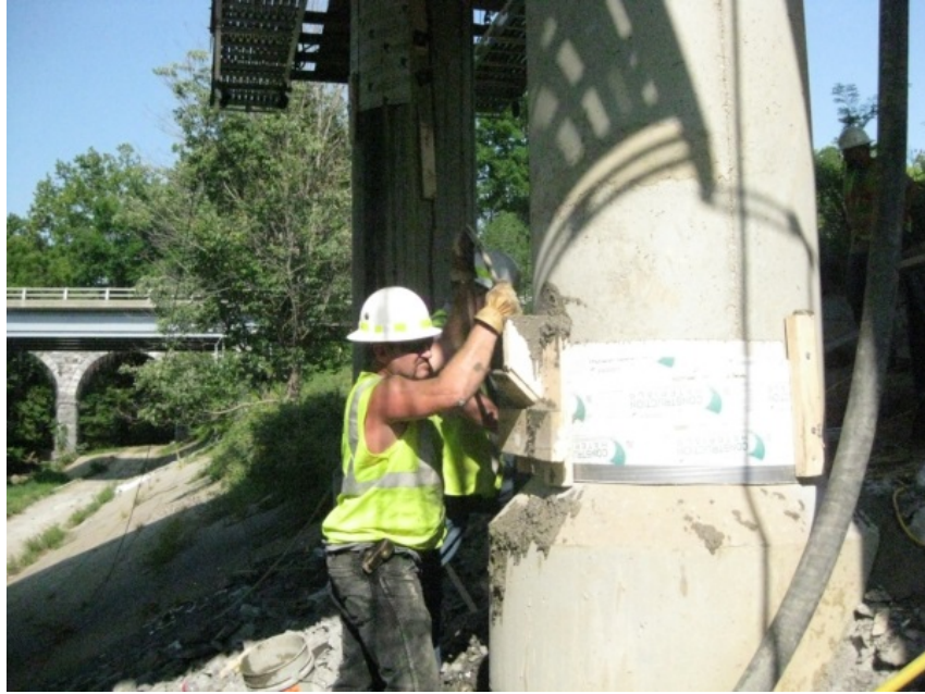
Figure 7. Column Being Consolidated With Internal Vibrator for I-81 Bridge
