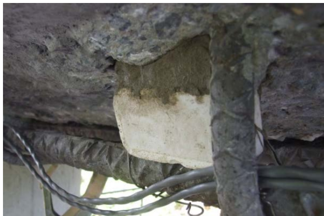
Figure 4. Exposed Steel and Anodes With Embedment Mortar for Route 712 Bridge
