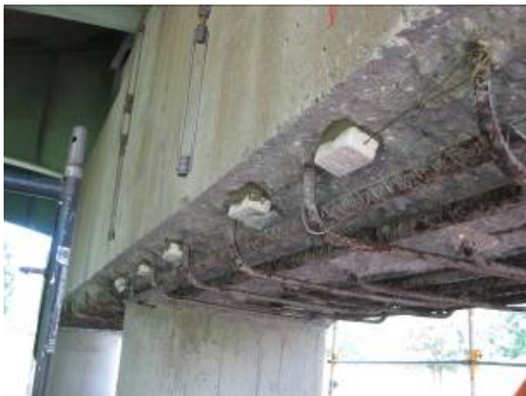
Figure 4. Exposed Steel and Anodes With Embedment Mortar for Route 712 Bridge
