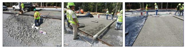
Figure 1. Construction Sequence at the Stringfellow Lot (L-R: Perforated Pipe Being Placed in the Loose Aggregate; Two-Directions of Rolling Compaction; Joints Being Placed)
