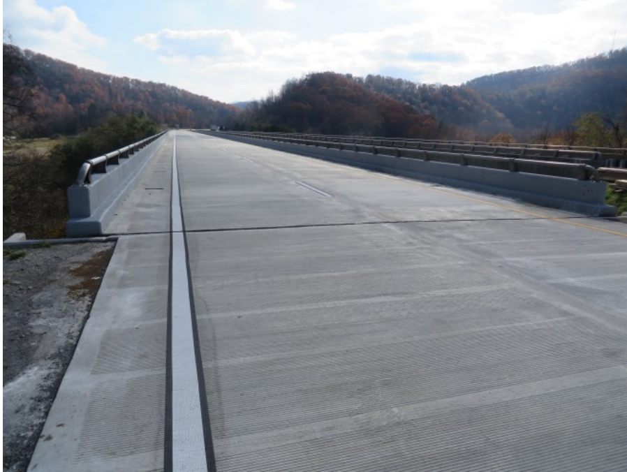
Figure 13. Finished Deck of Westbound Bridge
