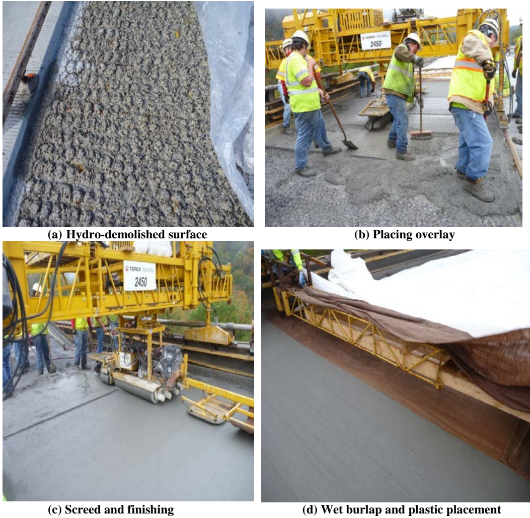
Figure 5. Overlay Placement Details for Dunlap Creek Bridge
