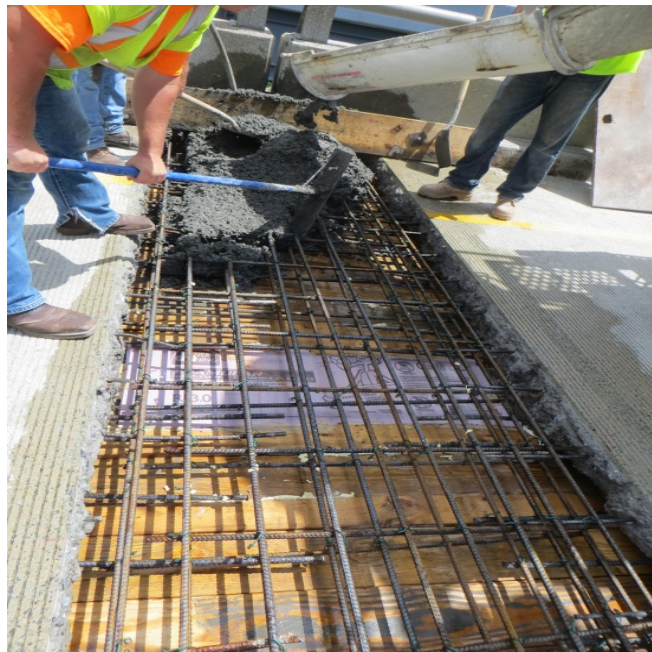
Figure 4. Concrete Placement in Closure Pours
