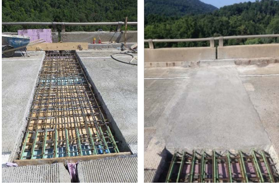
Figure 3. One Closure Pour Before Placement ( left ) and After Placement ( right )
