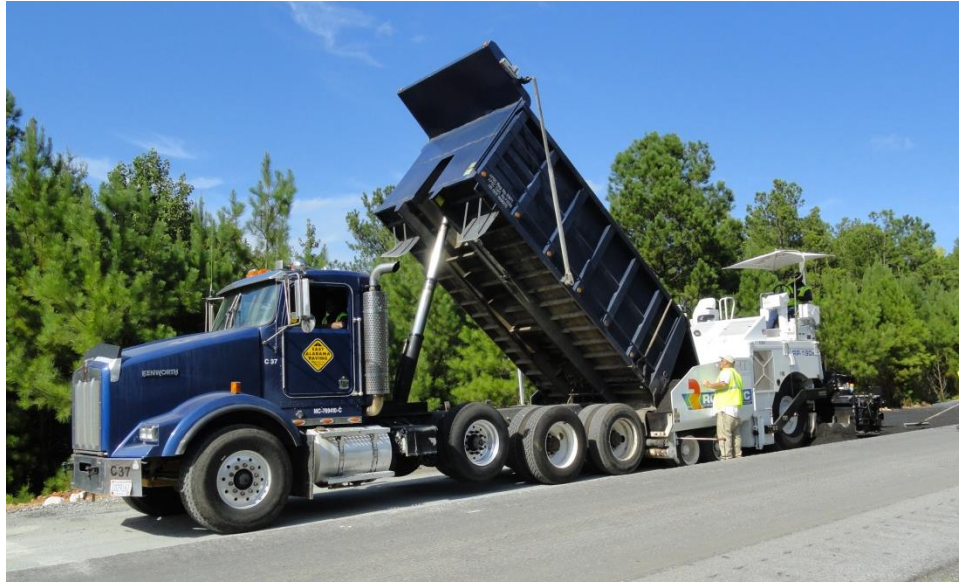
Figure 3. Transferring Cold Central Plant Recycled Material to an Asphalt Paver
