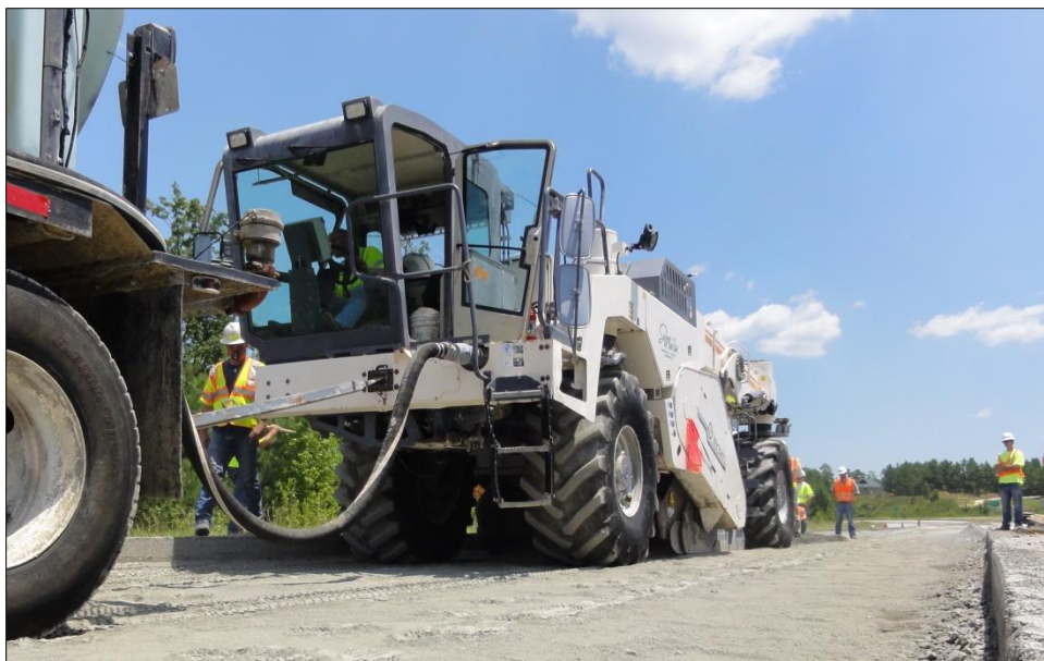
Figure 4. Full-Depth Reclamation Process in Section S12
