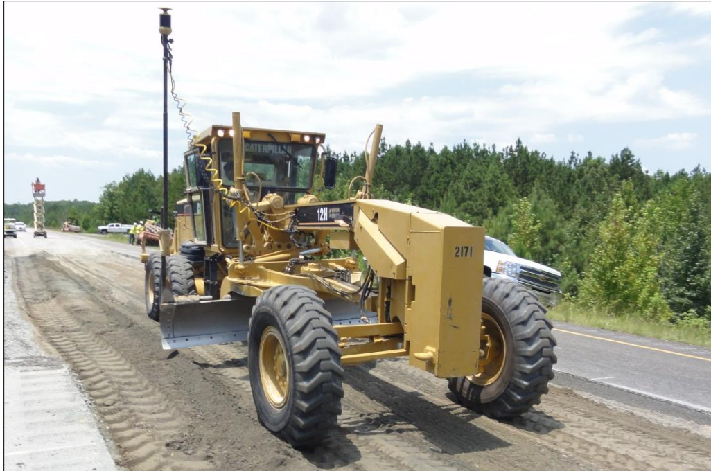
Figure 5. Shaping Cement-Stabilized Layer Using a Motor Grader
