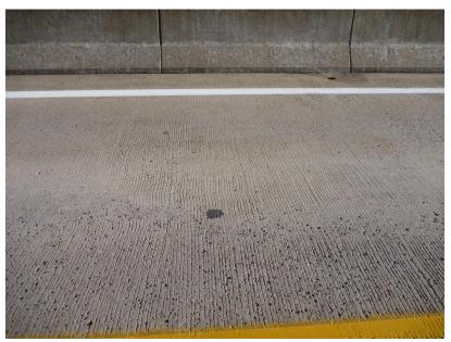
Figure 1. Lightweight Concrete Bridge Deck at Route 269 After 34 Years
