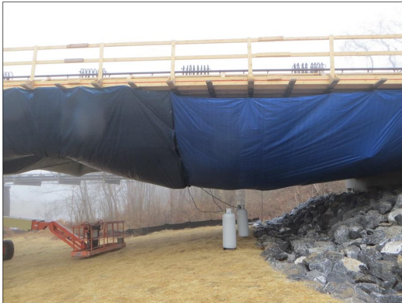
Figure 5. Concrete Protection and Heating System for Route 633 Covington
