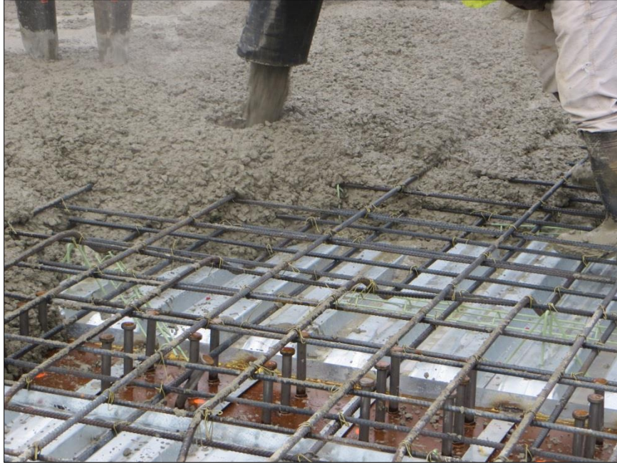
Figure 6. Concrete Mixture With SRA for Route 633 Covington
