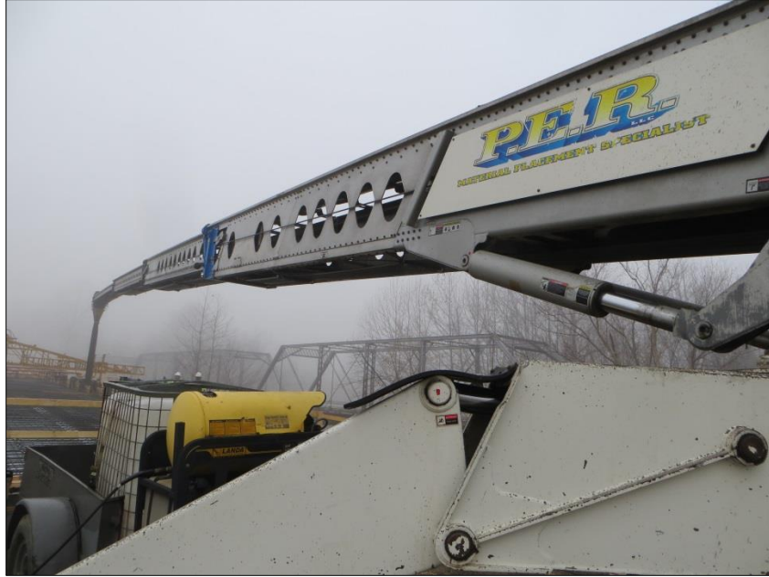
Figure 4. Conveyor Belt System for Placing Concrete for Route 633 Covington
