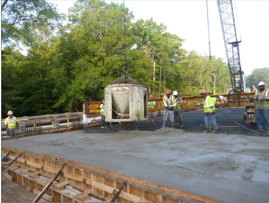
Figure 9. Concrete Placement Using a Bucket for Route 600 Herring Creek
