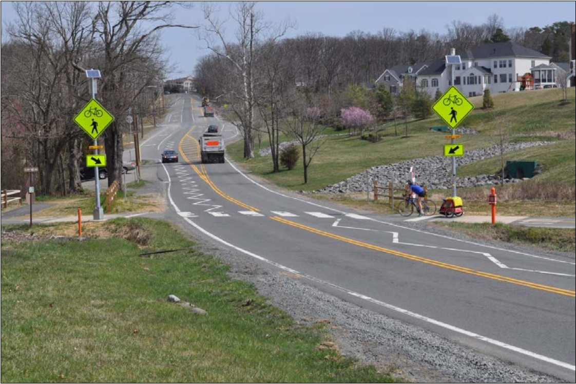
Figure 5. RRFBS and Signage at W&OD Trail Crossing
