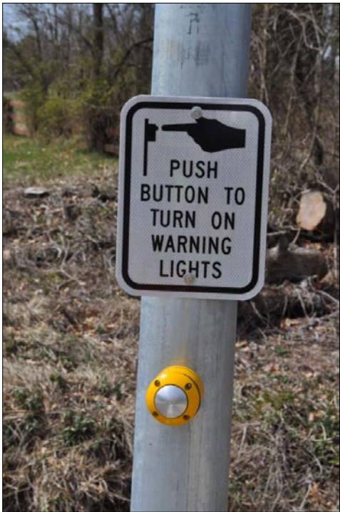
Figure 6. RRFB Push Button and Sign
