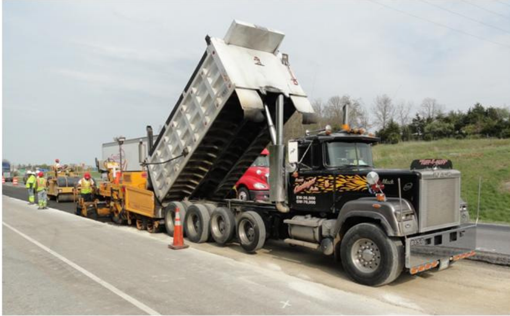
Figure 5. Paving the Cold Central-Plant Recycling Material
