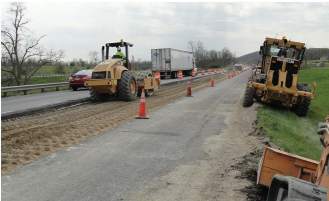
Figure 3. Compaction of Full-Depth Reclamation Layer
