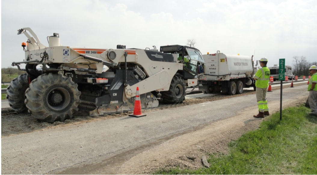
Figure 2. Full-Depth Reclamation Process Used in Right Lane
