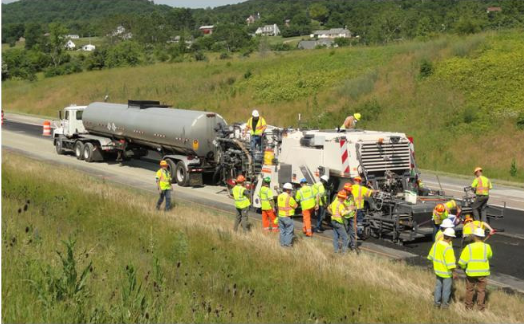
Figure 6. Cold In-Place Recycling Process Used in Left Lane
