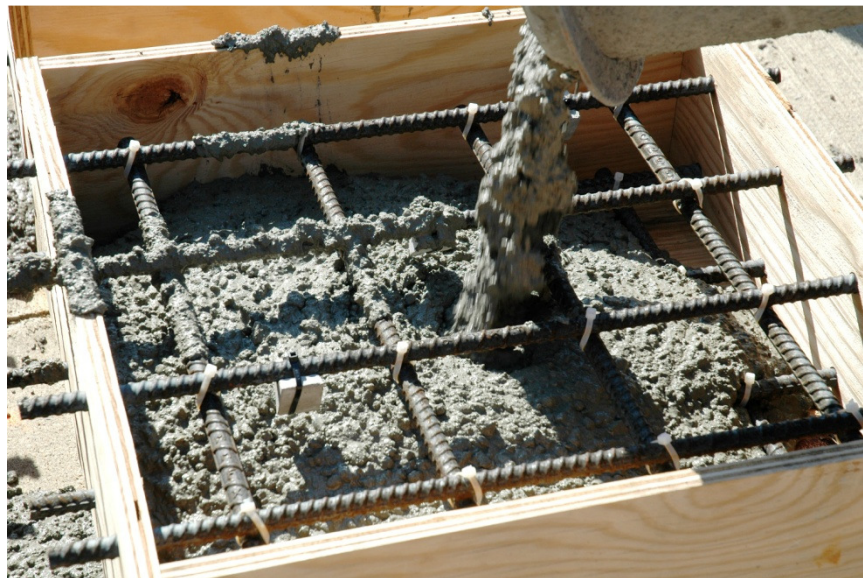
Figure 9. Placement of SCC in Sample. SCC = self-consolidating concrete.
