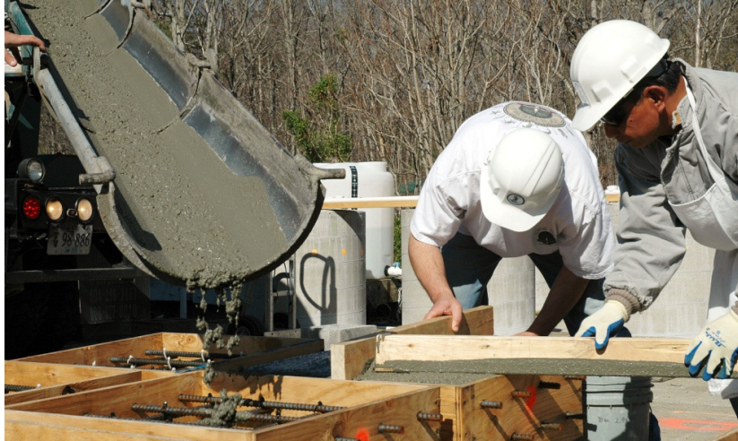
Figure 10. Striking Off of SCC. SCC = self-consolidating concrete.
