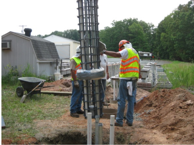
Figure 7. Cage is lowered into mold in ground.
