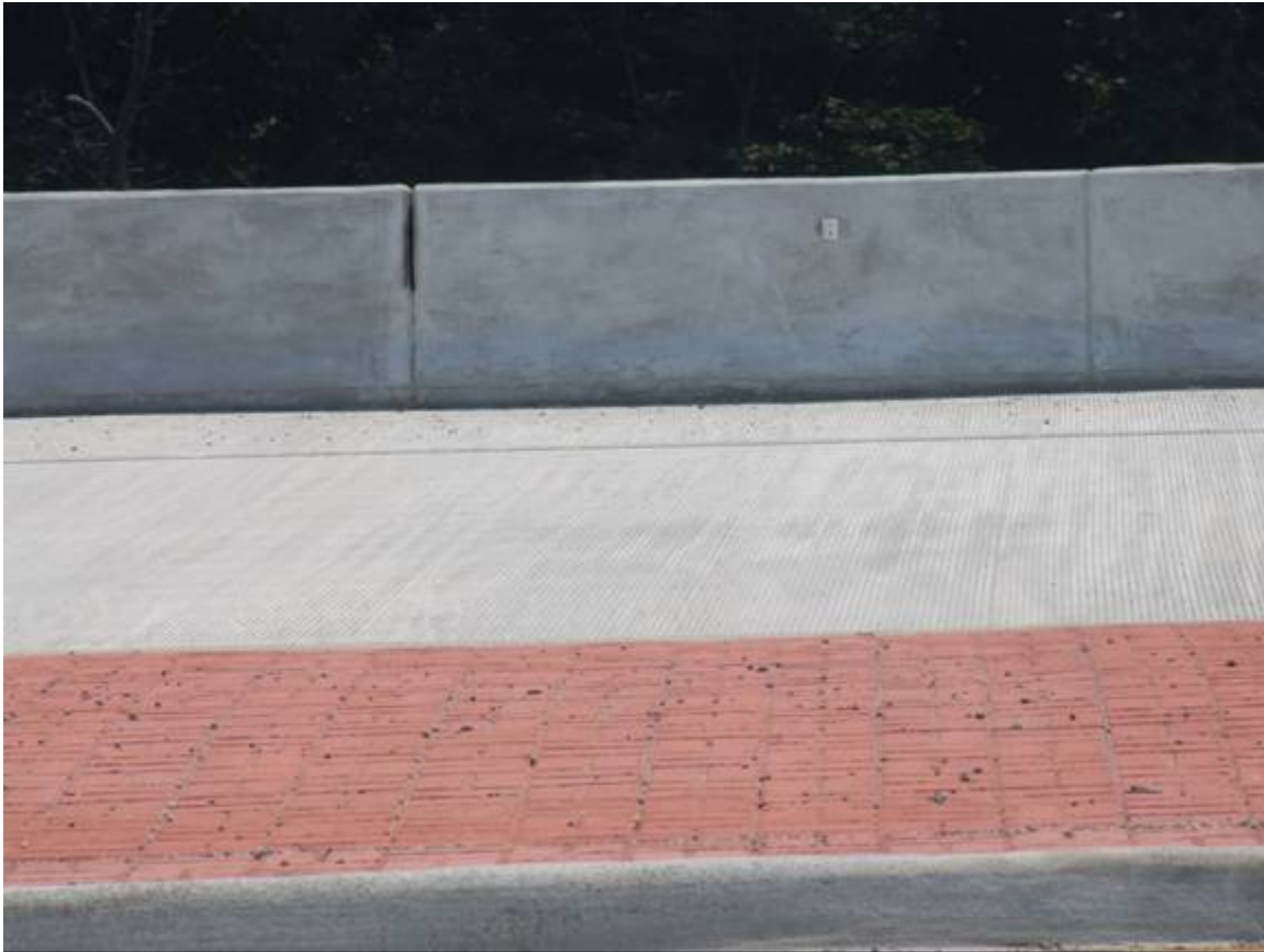
Figure 25. Northbound (MMFX 2) Raised Median and Deck Image
