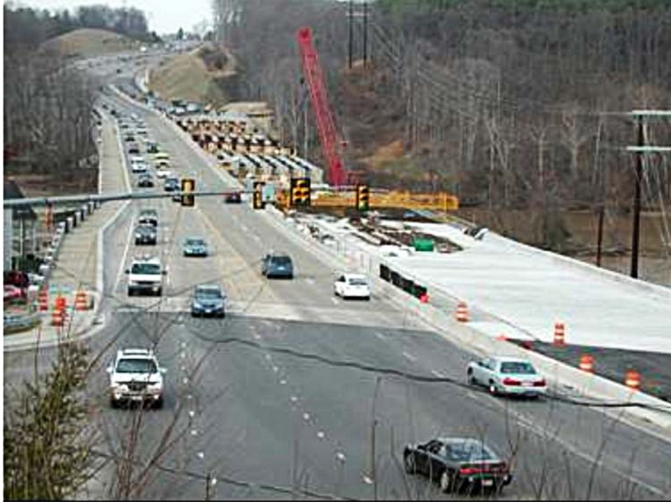
Figure 7. Traffic Configuration Before Southbound (ECR) Deck Sealing Operations
