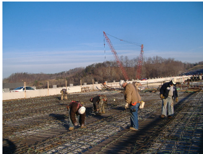
Figure 34. Walkways Not Required Over MMFX 2
