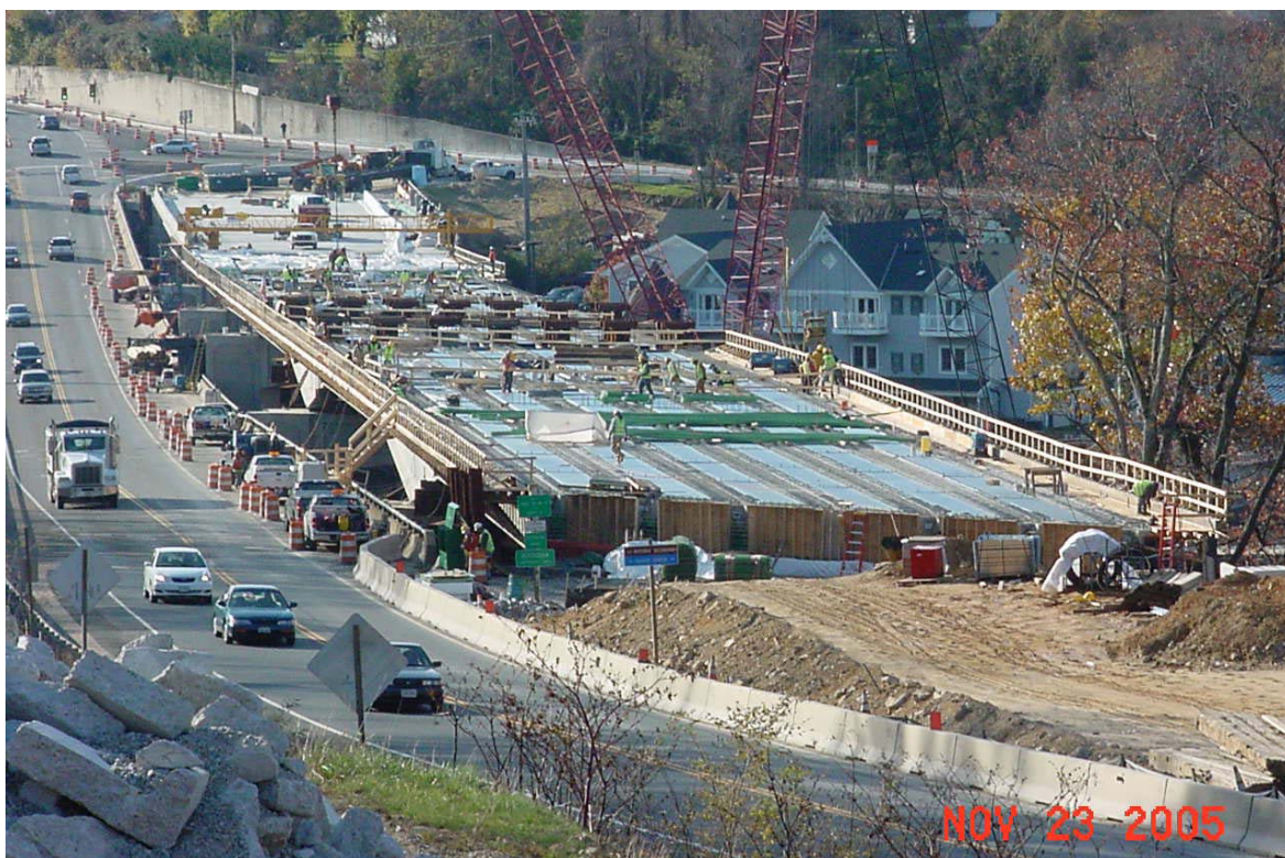
Figure 2. ECR Placement in Southbound Lane
