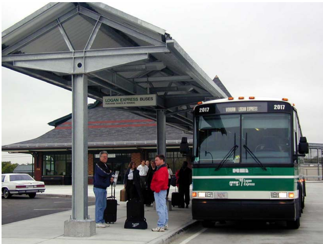
Figure 3. Logan Express Bus Terminal at Woburn, Massachusetts. Courtesy of Douglas Wheaton, Massachusetts Port Authority.
