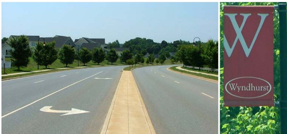
Figure 2. Wyndhurst Neighborhood (Enterprise Drive, Section Adjacent to Figure 1)
