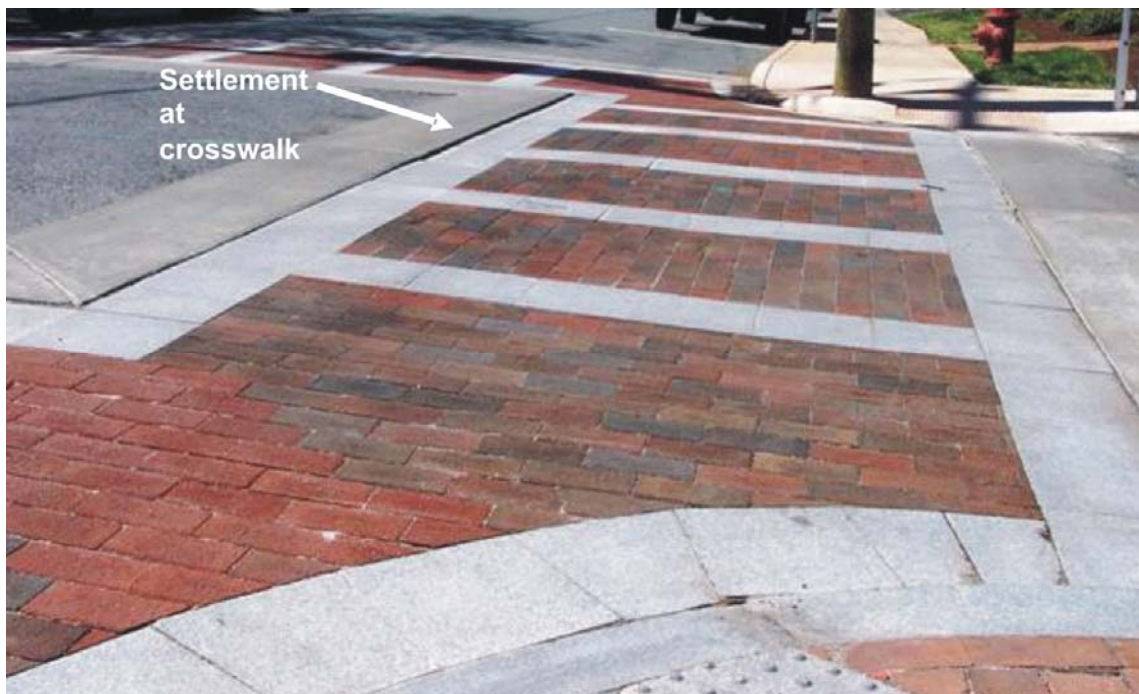
Figure 1. Example of Paver Crosswalks at Charlottesville's Court Square
