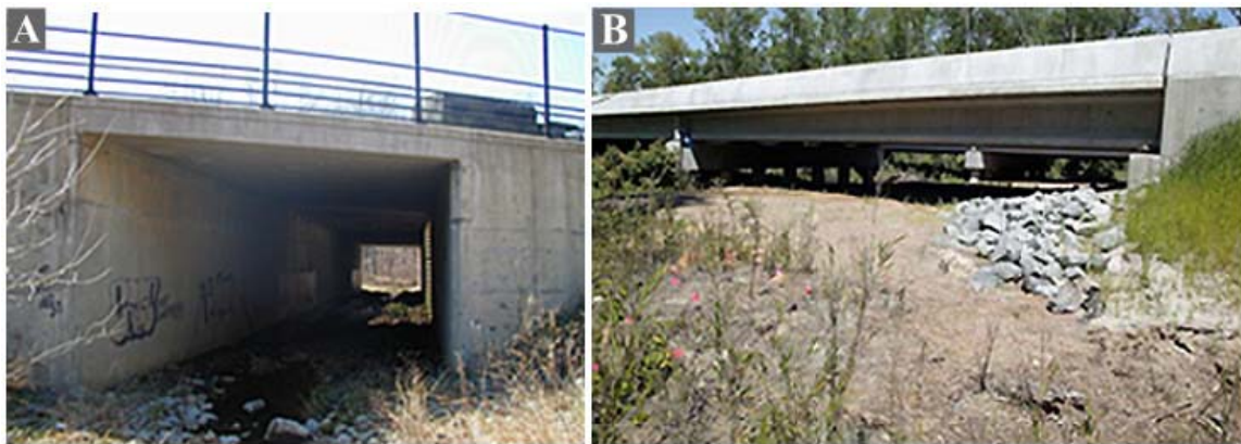
Figure 3. (A) A box culvert, 15 x 20 ft, in Fairfax County, Virginia. (B) A 984-ft bridge over a wetland in Chesapeake, Virginia, modified with a “boardwalk” to provide a dry passageway for wildlife.
