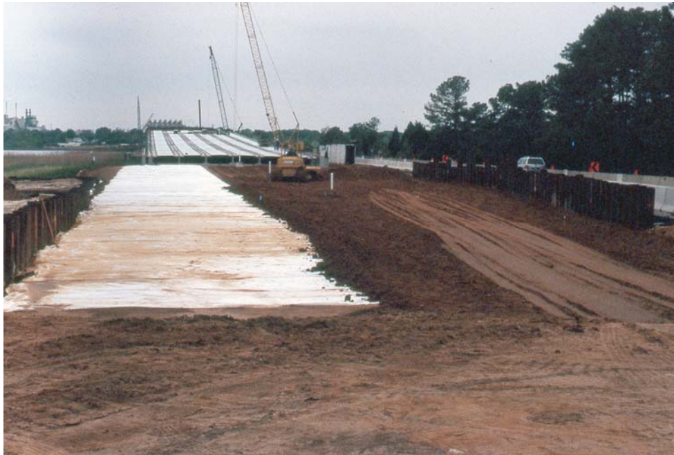
Figure 8. Reinforcing Fabric and Settlement Pipes
