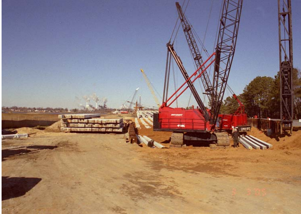
Figure 4. Pile Installation
