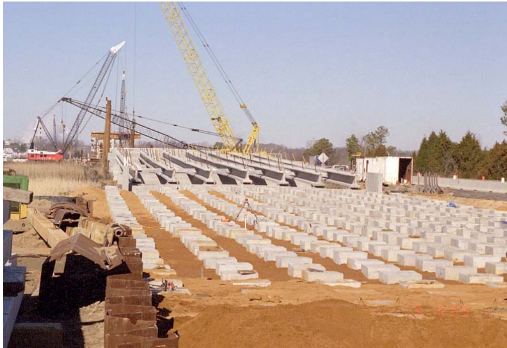
Figure 5. Installed Pile Caps
