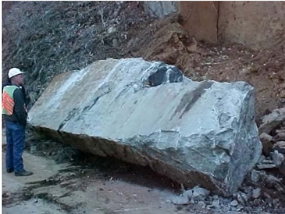
Figure 1. Rockfall at Route 56 Near Crabtree Falls, Nelson County (February 2001)
