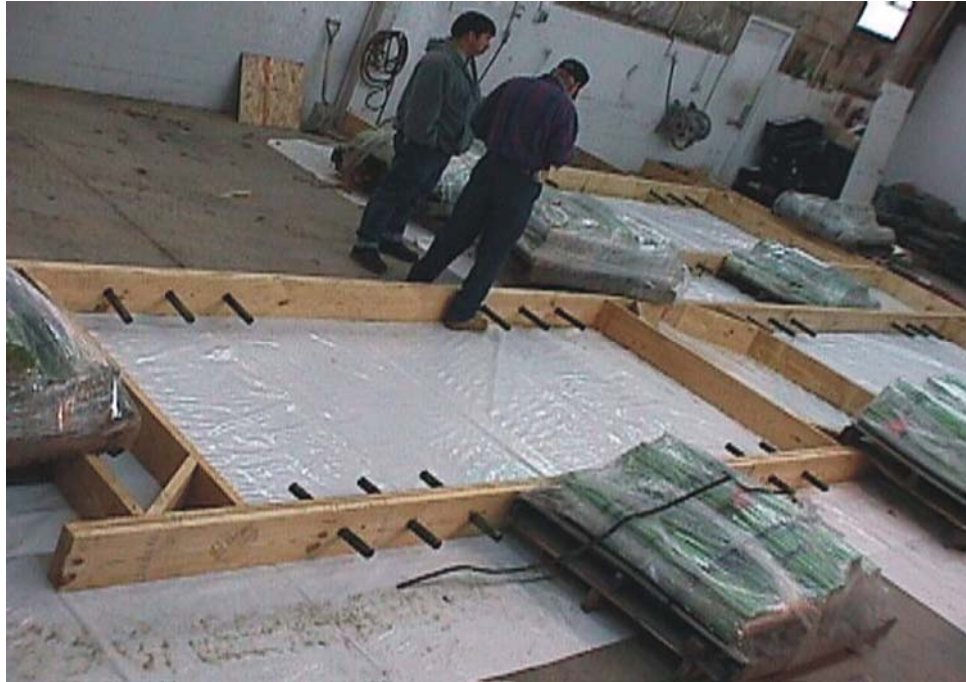
Figure 2. Precast Patch Fabrication With Cast-In Dowels
