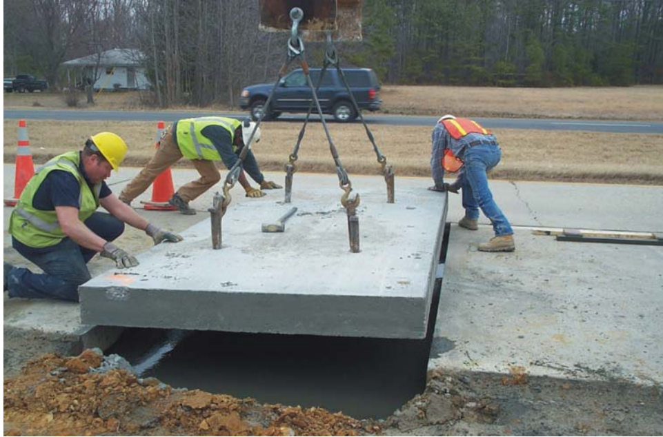
Figure 5. Placement of Precast Slabs
