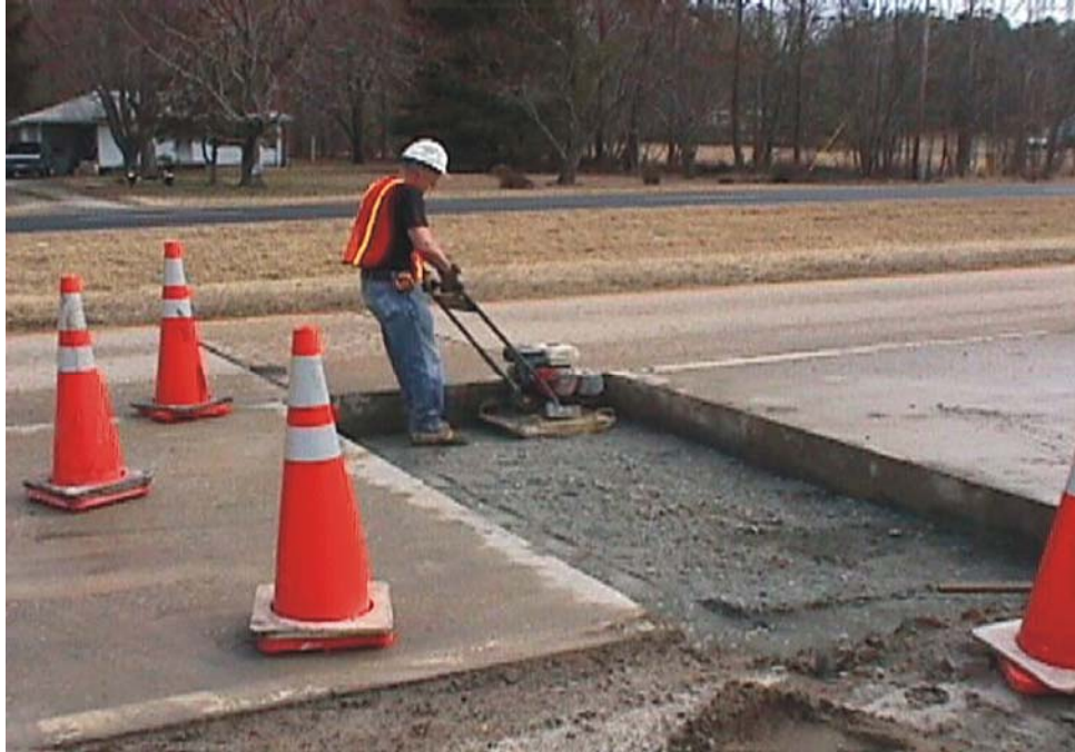
Figure 3. Recompaction of Existing Base
