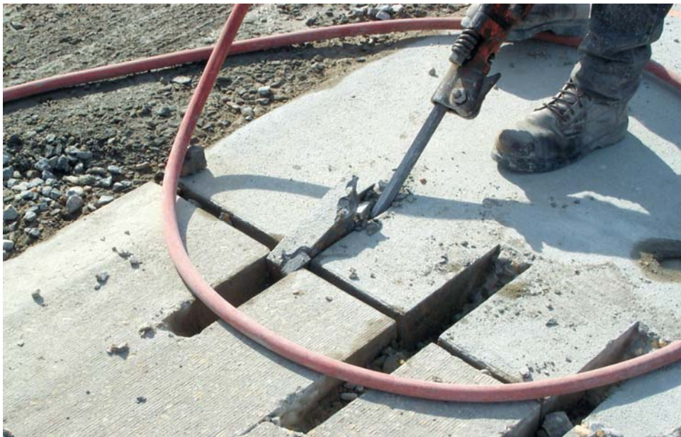
Figure 6. Dowel Bar Retrofit
