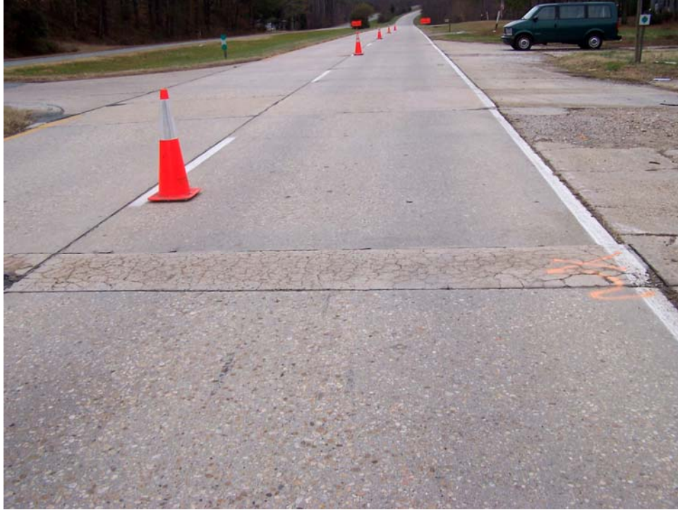
Figure 1. Pavement Condition Before Precast Patching Installation
