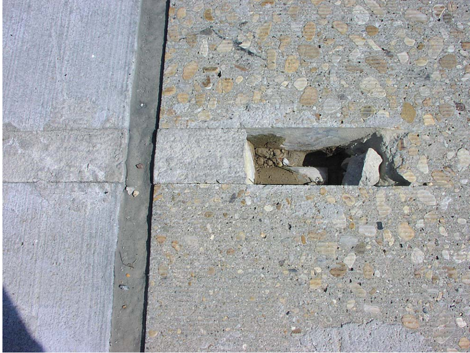
Figure 10. Exposed Dowel
