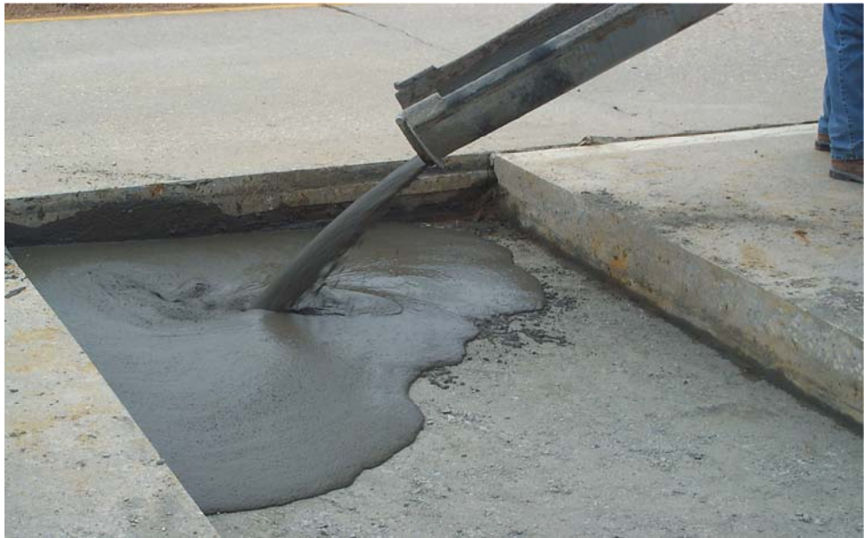
Figure 4. Flowable Fill for Leveling
