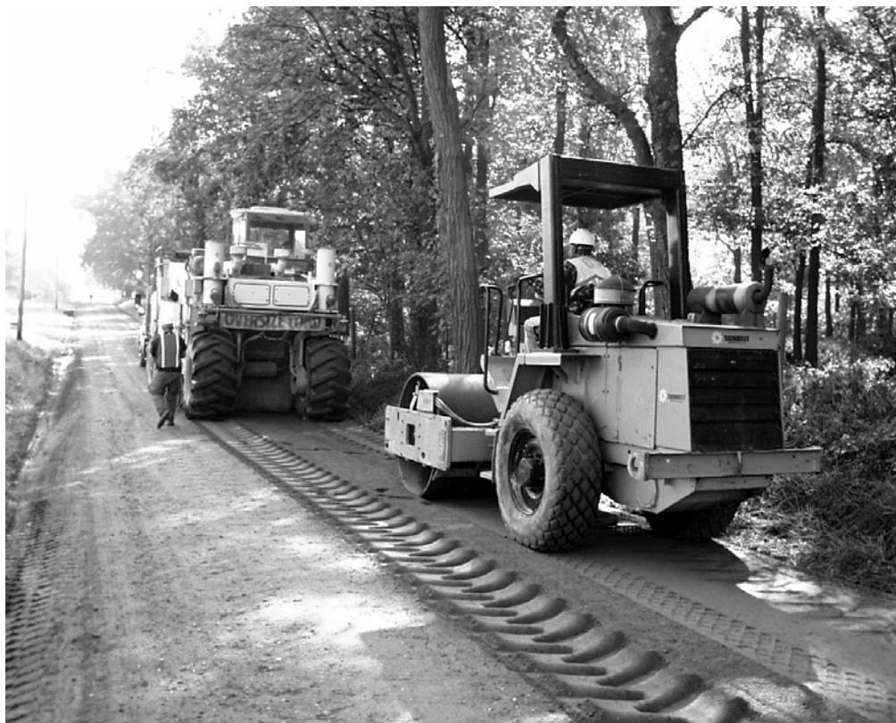
Figure 4. Material Compaction Following Roadbed Manipulation
