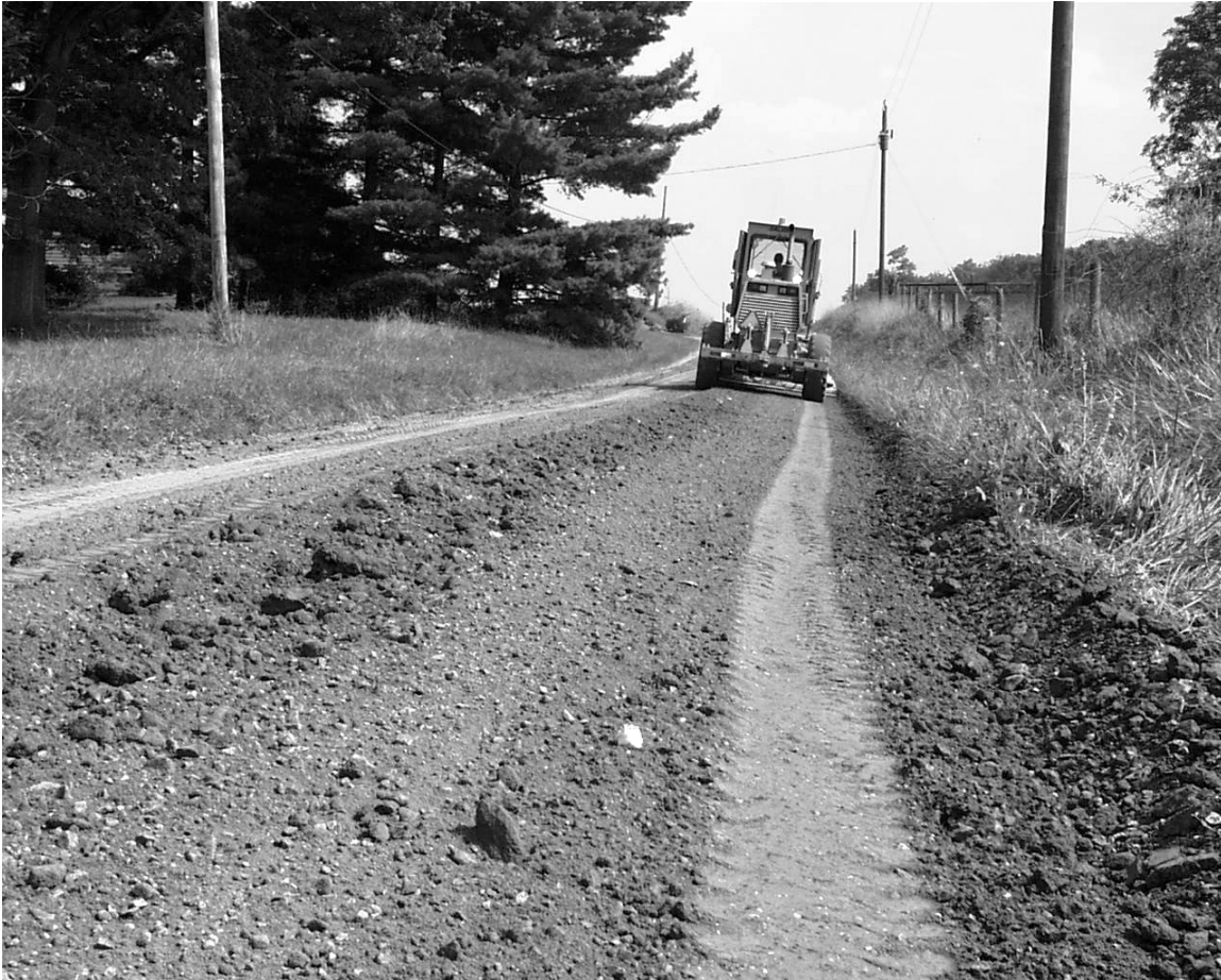
Figure 3. Roadbed Preparation Prior to Manipulation
