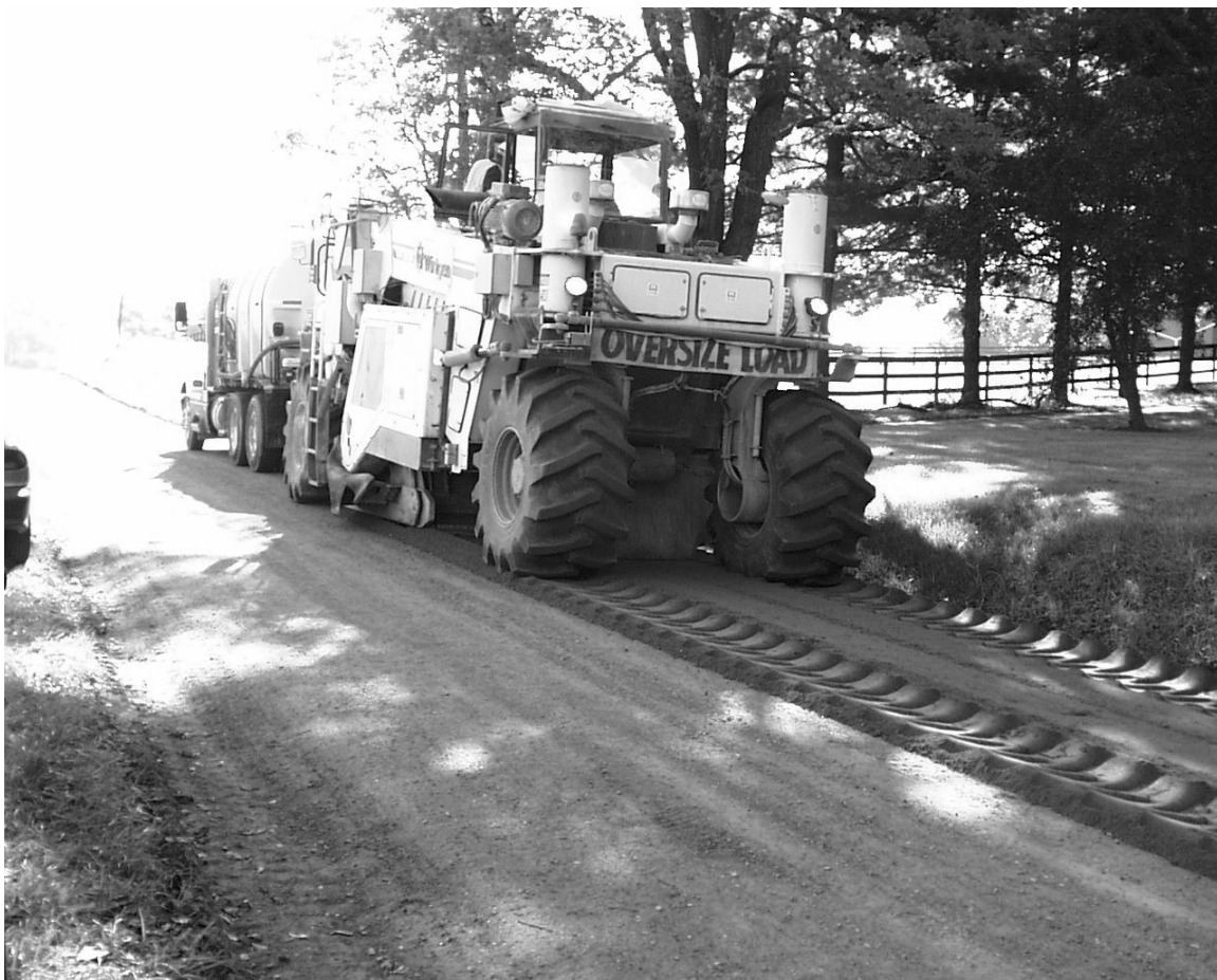
Figure 2. Gravel Road Stabilization with Wirtgen WR 2500 Full-Depth Reclaimer
